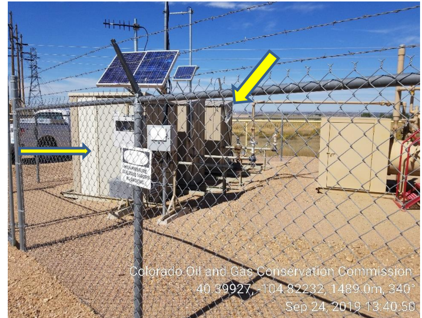
Photo 14: Disconnected gas meter houses
