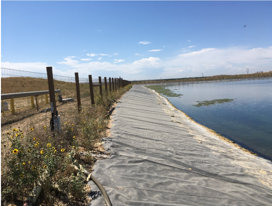
Pit. Photo looking south. Liner in good condition.
