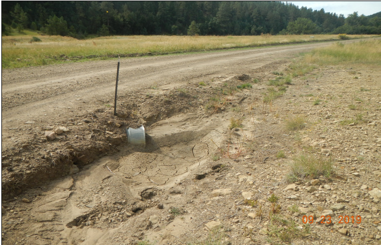
Photo 1. The culvert along the main road has partially filled in with sediment. It appears to have been cleaned out since the previous inspection but requires ongoing maintenance.
