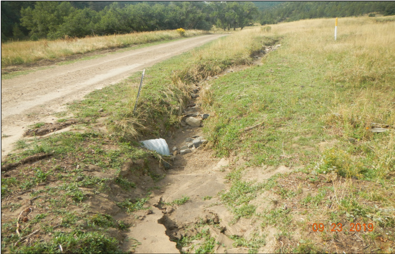
Photo 2. The culvert has been cleaned out from sediment buildup. Lat/Long:37.02425,-104.82919
