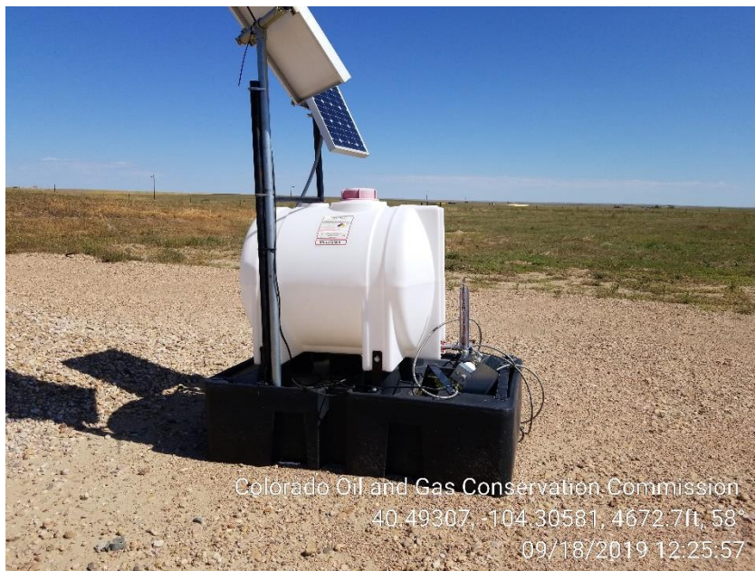
Photo 3 – Unused Methanol Tank/Pump on the Northeast side of location
