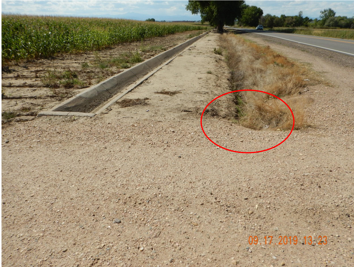
Photo 2. Photo taken from the well location entrance point, facing West. Photo illustrates the Operator has failed to remove the culvert. There is an access point for this crop field ~600 feet to the west of this point. This access point is no longer in use and was used for oil and gas operations.
