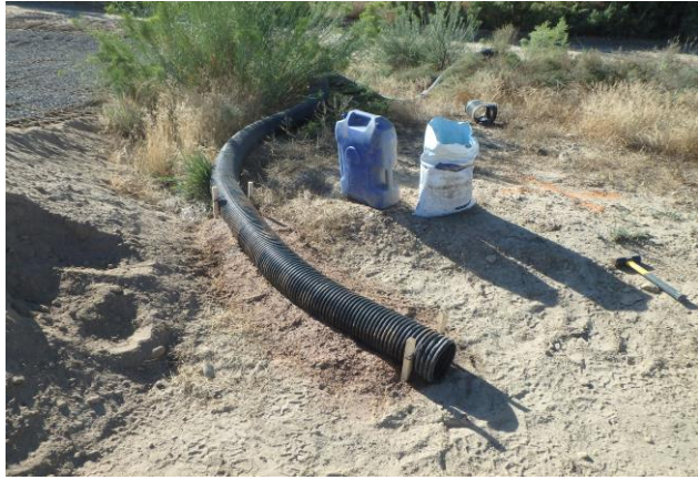
Installing Flex Pipe Outlet
