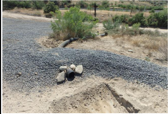
Flex Pipe Outlet Installed
