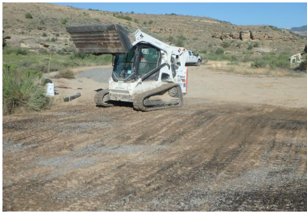
Compacting Earthen Berm and Pad Entrance
