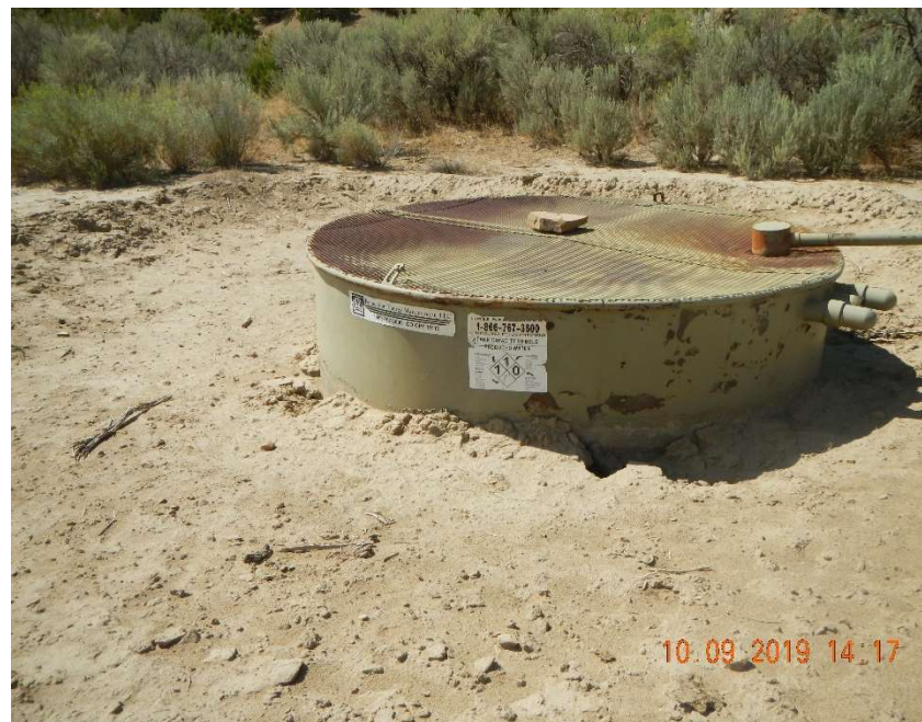
Photo #8 – View of the 60 bbl produced water tank.
