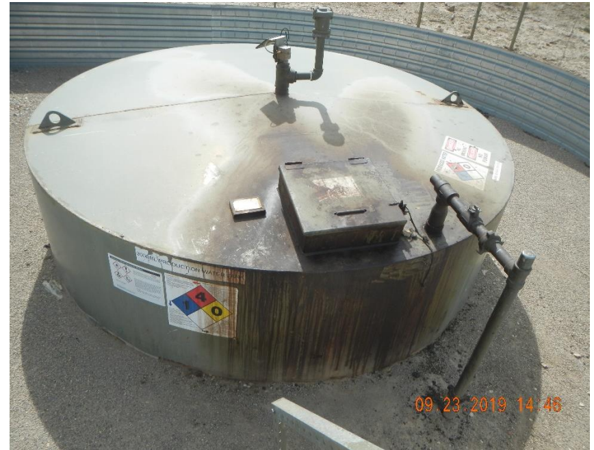
Labels on 200 bbl tank needed cleaned.
