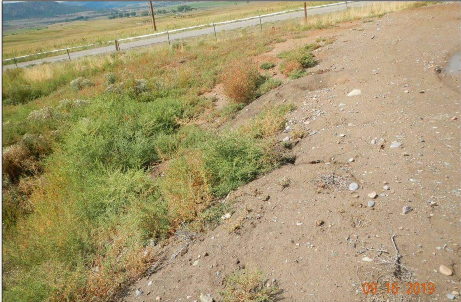
Photo 2. View of the southern fill slope facing westward. Slope is not stabilized as weedy kochia is preventing desirable vegetation establishment and bare soils are eroding.
