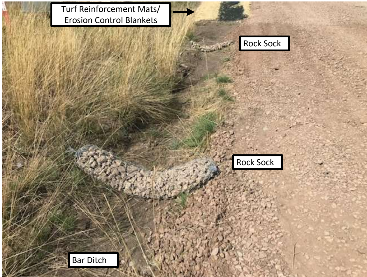
Photo 2: In the undisturbed portion of the bar ditch, (3) sets of rock socks were installed up gradient of the turf reinforcement mats to filter out sediment. Rock socks are made from 1" chicken wire filled with gravel.
