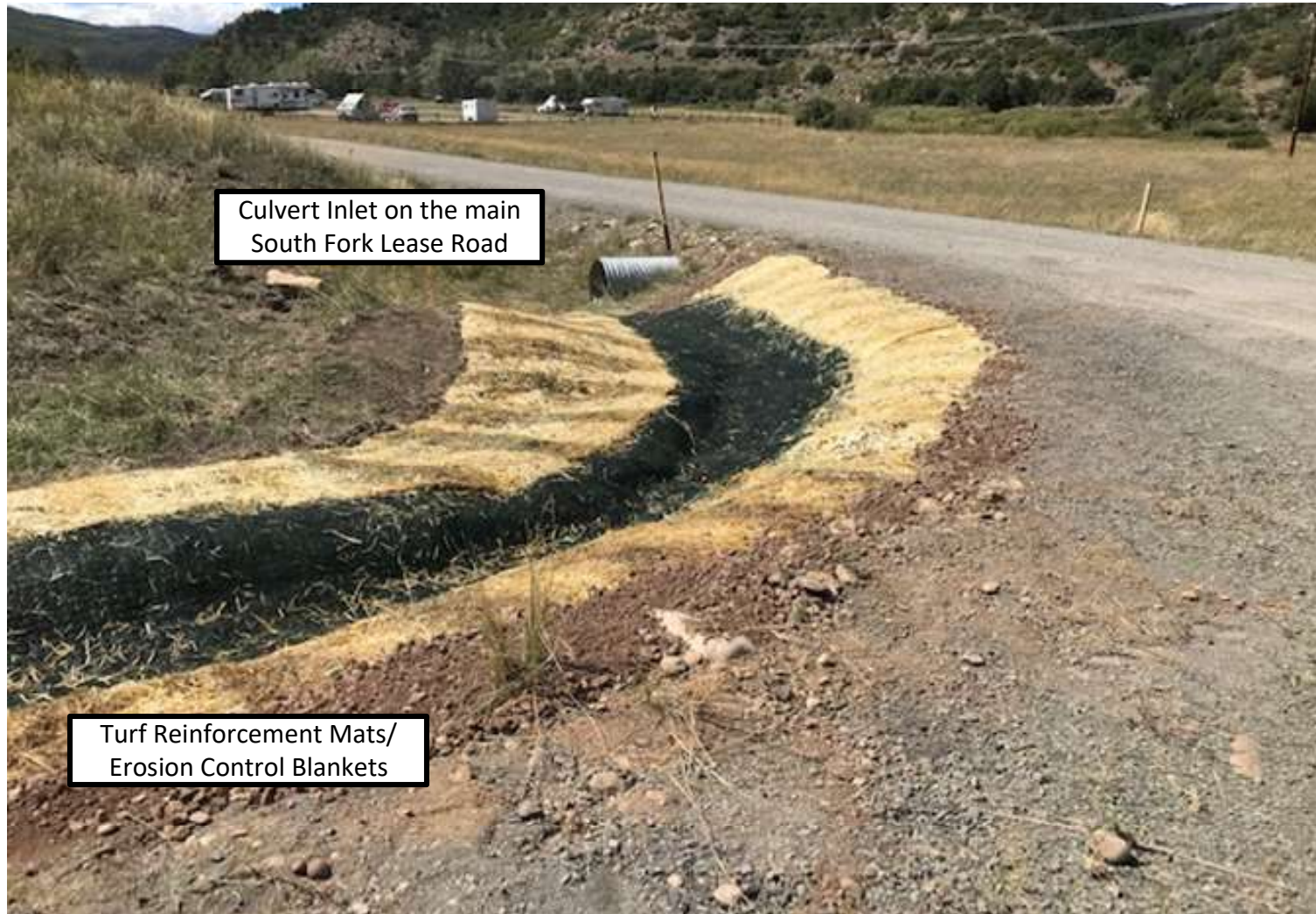
Photo 4: Turf reinforcement mats were installed in the bar ditch to reduce the potential for erosion. Erosion control were installed where the soil was disturbed on both sides of the bar ditch to reduce the potential for sediment discharge. An approved CPW seed mix was used to establish vegetation.
