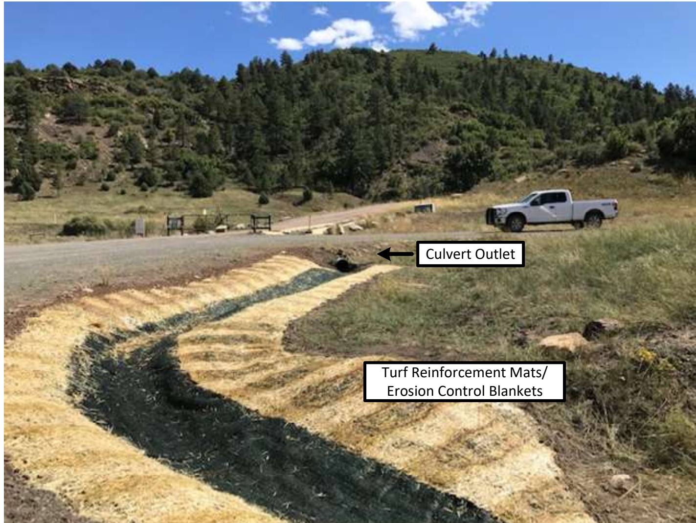
Photo 3: On Little Bingham facing toward the entrance to AC 20-01. The bar ditch was dominated to direct run off to the culvert inlet on the South Fork Lease Road. Turf reinforcement mats were installed in the bar ditch and erosion control were installed where the soil was disturbed on both sides of the bar ditch. An approved CPW seed mix was used to establish vegetation.
