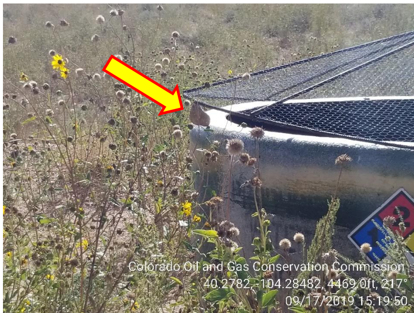
Photo 9 – Rock is wedged between vault and netting, creating a potential opening for Wildlife.
