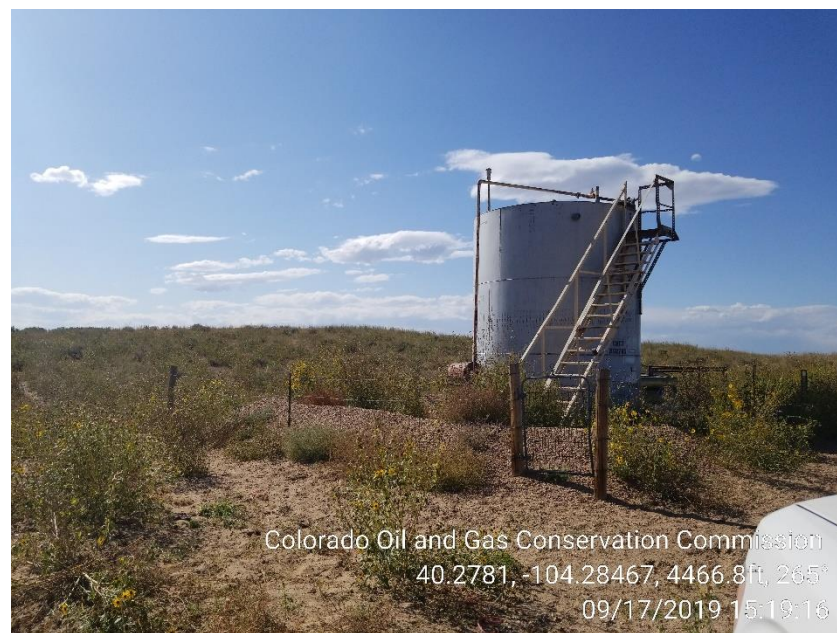
Photo 2 – Tank Battery; weeds actively growing in and around berm
