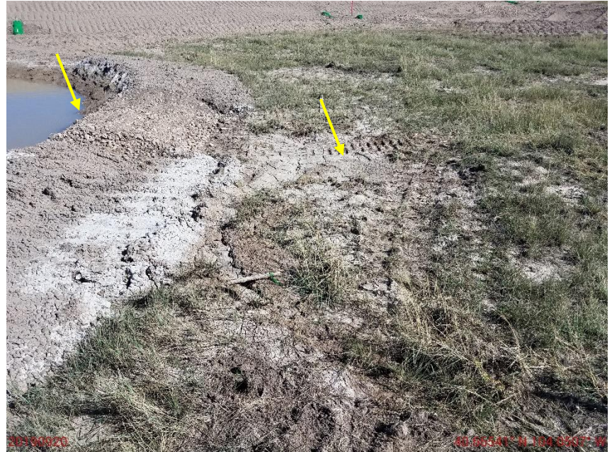
Photo 4: Photo shows area of the sediment trap BMP that appears to have failed resulting in sediment laden stormwater discharge
