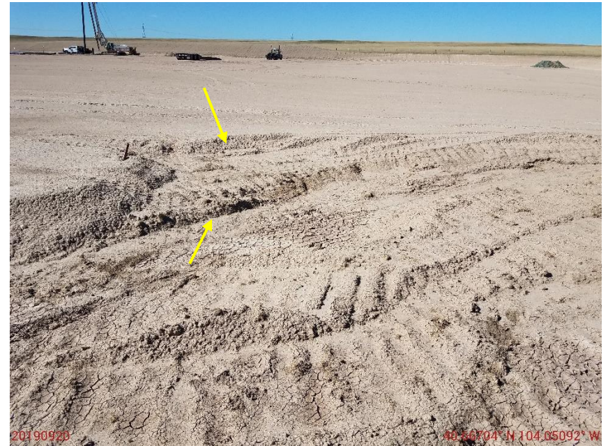
Photo 14: Photo taken from the east end of the location. Photo shows area where pad meets the perimeter diversion ditch. Photo shows insufficient BMPs in place to stabilize soils and location.
