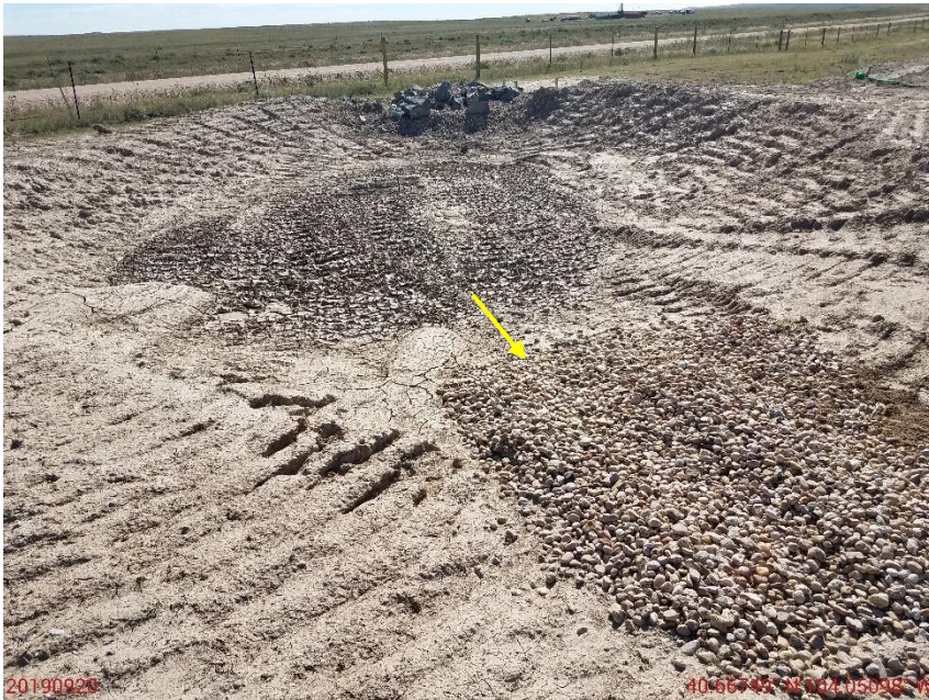
Photo 17: See comments under photo 15. Photo also shows operator has installed rock aggregate along inlet.
