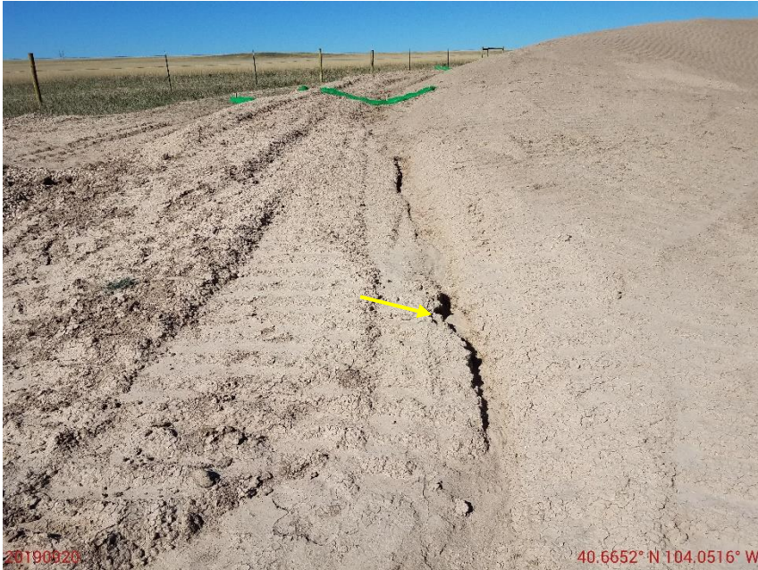
Photo 25: Photo taken from the stormwater ditch on the south end of the location. Photo shows erosion degradation within ditch.
