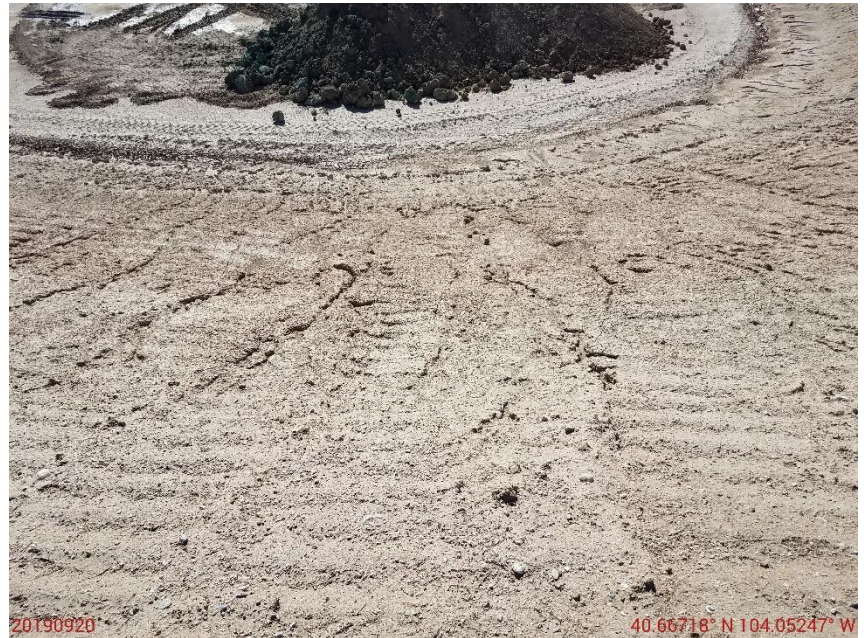
Photo 18: Photo taken from the northwest end of the location. Photo shows erosion degradation on slopes due to insufficient stormwater and erosion control BMPs.
