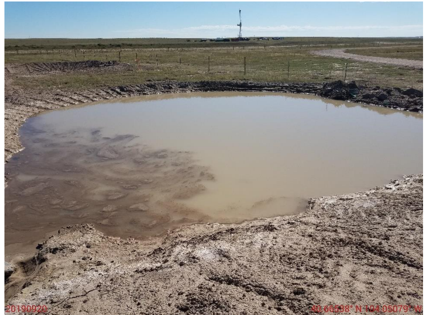
Photo 2: Photo of sediment trap on the south end of the location. It appears BMP is sufficient in size to mitigate runoff on the location. However (though repaired) it appears that areas of the trap had failed resulting in sediment laden stormwater discharge. See photos 4-6.
