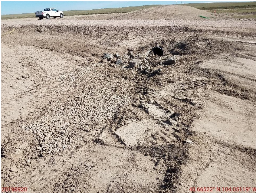
Photo 29: Photo taken from the culvert on the south end of the location. Photo shows sufficient outlet protection has not been installed above culvert outlet. Sediment is also beginning to fill culvert and rip-rap; maintenance advised.
