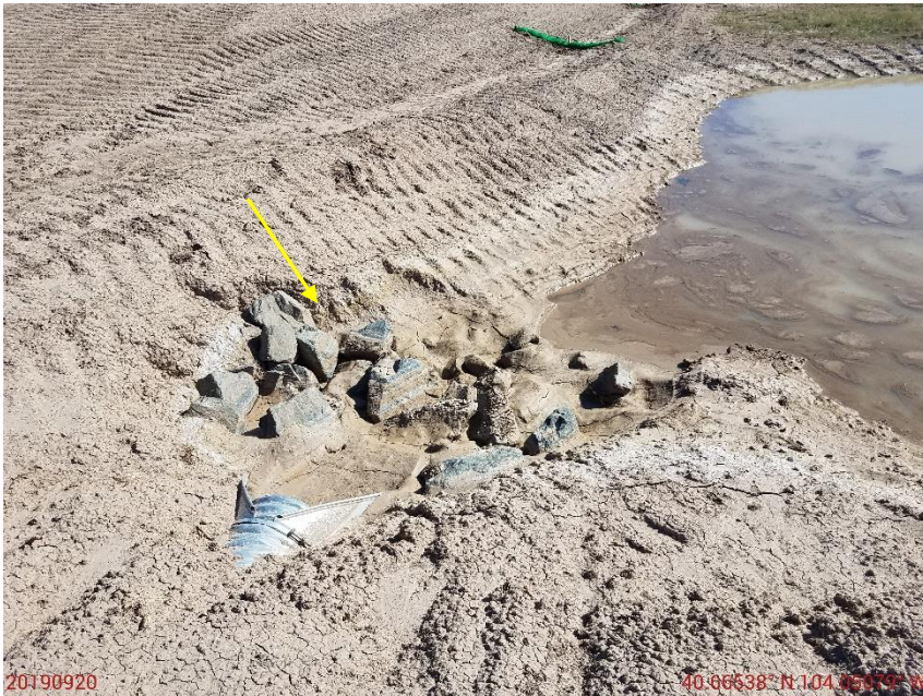
Photo 1: Photo taken from the culvert/sediment trap on the south end of the location. Photo shows sufficient outlet protection has not been installed above culvert outlet. Culvert outlet/sediment trap inlet has filled with sediment
