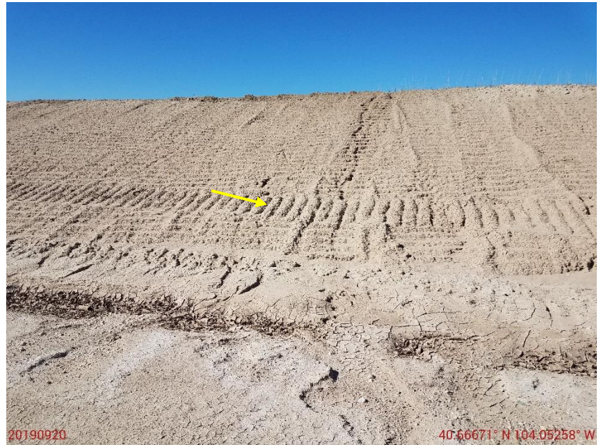
Photo 20: Photo taken from the northwest end of the location, facing west. Photo shows operator has not installed stabilization controls on slopes in accordance with good engineering practices. Operator has installed tracking along the contour of the slopes rather than up and down. This has resulted in the facilitation of rill erosion on the slopes.
