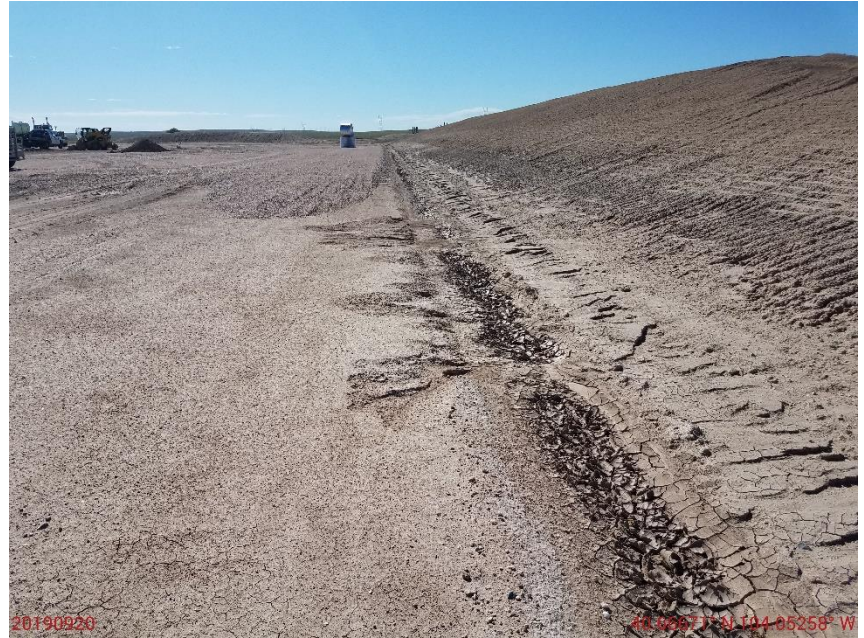
Photo 22: Continued from photo 20. Photo shows sediment deposition due to stormwater erosion on slopes.
