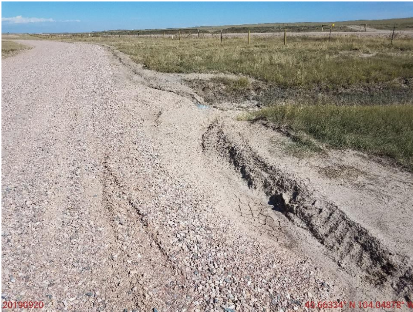
Photo 33: Photo taken from cattle guard along access road. Photo shows insufficient outlet protection at culvert. Erosion degradation evident.
