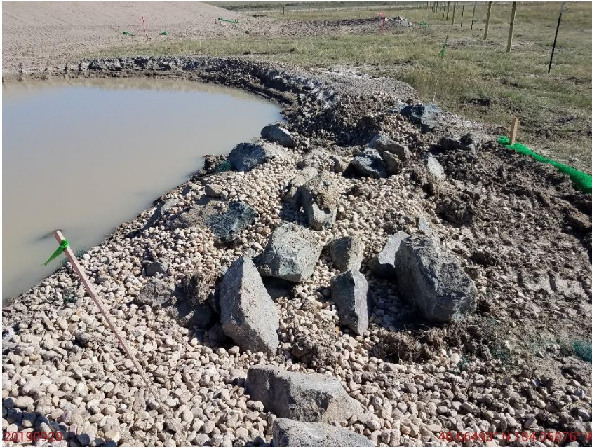
Photo 7: Photo taken from the outlet at the sediment trap. Operator appears to have installed the outlet at the same elevation as the adjacent berms, and constructed in such a manner to dam stormwater rather than reducing velocity, trapping excess sediment and allow for sediment laden-free stormwater discharge from the trap. BMP has not been constructed with good engineering practices.
