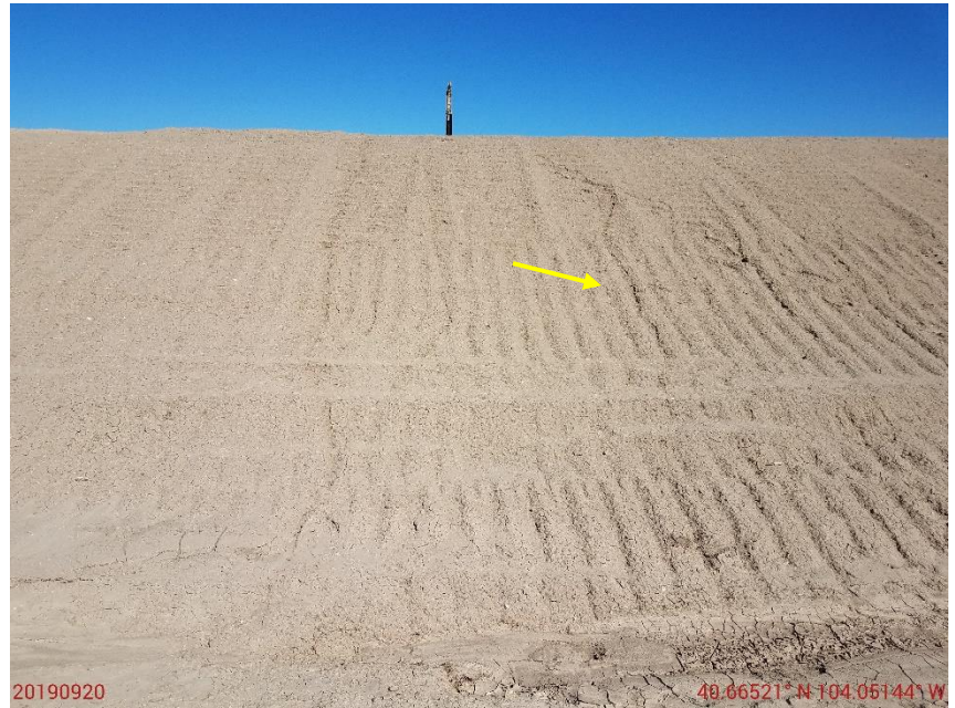
Photo 28: Photo taken from the topsoil stockpile on the southwest end of the location. Photo shows operator has not installed stabilization controls on slopes in accordance with good engineering practices. Operator has installed tracking along the contour of the slopes rather than up and down. This has resulted in the facilitation of rill erosion on the slopes.
