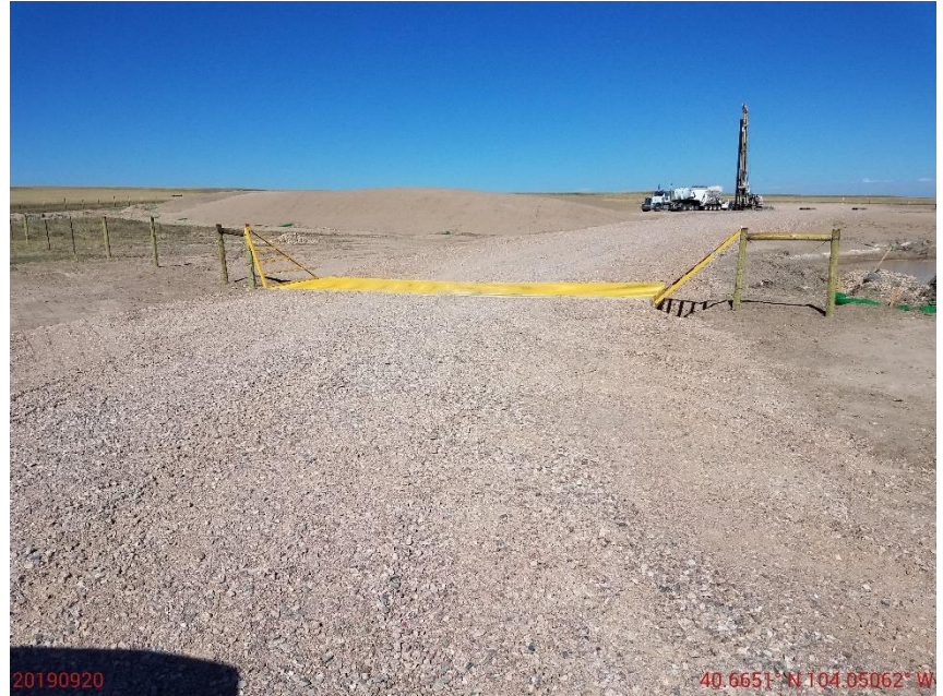
Photo 32: Photo taken from the access road south of the location, facing north. Photo of cattle guard. Insufficient tracking BMPs on location and/or access road.
