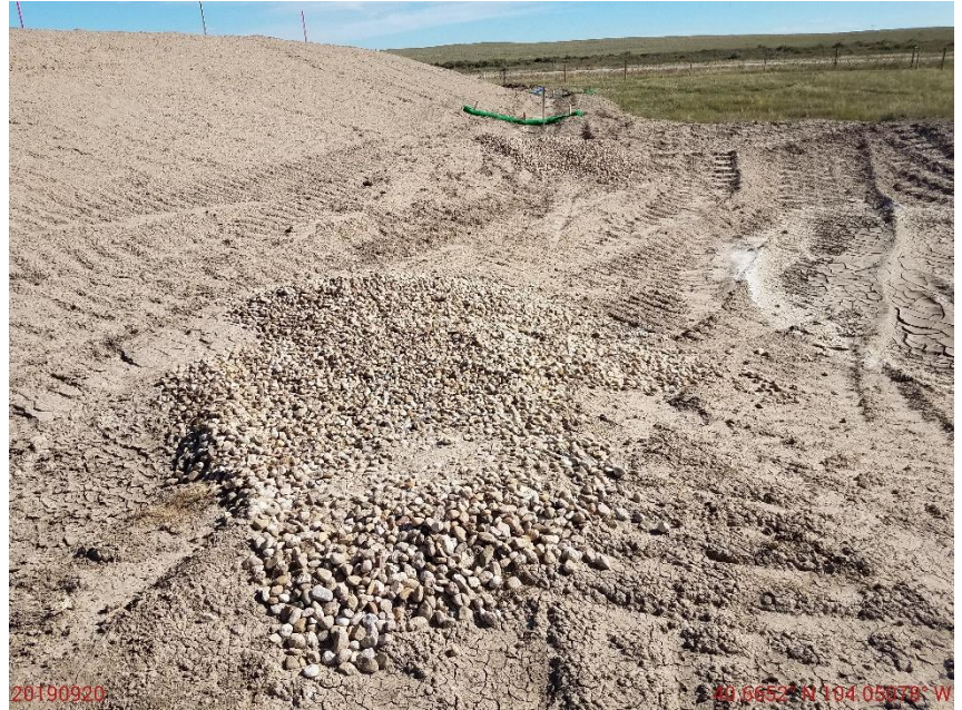
Photo 8: Photo taken from the sediment trap on the southeast end of the location. Photo shows operator appears to have installed rock aggregate as inlet protection.
