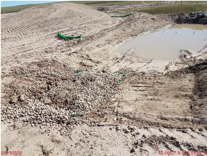
Photo 23: Photo taken from the sediment trap on the southwest end of the location. Photo shows operator has installed inlet protection on a portion of the inlet. BMP does not appear to be sufficient as erosion degradation is evident.
