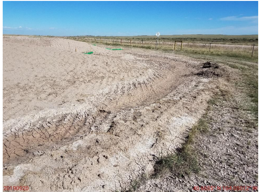
Photo 10: Photo of diversion ditch on the southeast end of the location. Erosion degradation on the slopes have resulted in sediment deposition within ditch. Maintenance required.
