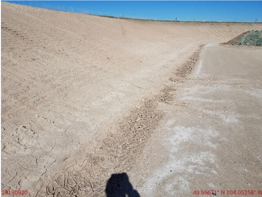
Photo 21: Continued from photo 20. Photo shows sediment deposition due to stormwater erosion on slopes.
