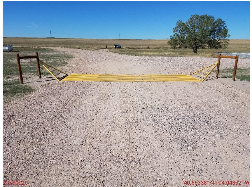
Photo 36: Photo taken from the access road south of the location, facing west. Photo of cattle guard. Insufficient tracking BMPs on location and/or access road.
