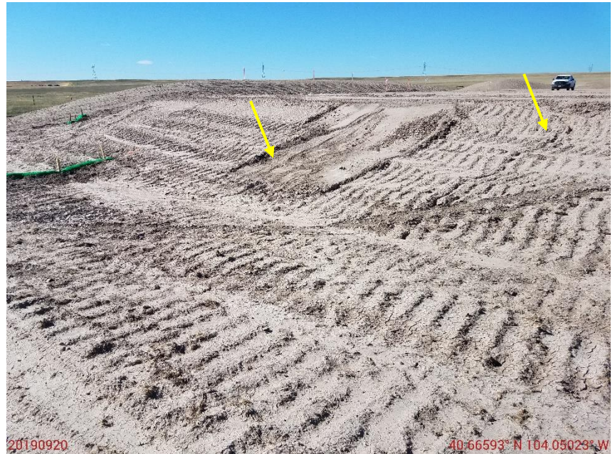
Photo 12: Photo taken from the southeast end of the location, facing west. Photo shows area where stormwater erosion appears to have degraded the slopes. Operator appears to have repaired the erosion. However, photo also shows operator has not installed stabilization controls on slopes in accordance with good engineering practices. Operator has installed tracking along the contour of the slopes rather than up and down. This has resulted in the facilitation of rill erosion on the slopes.
