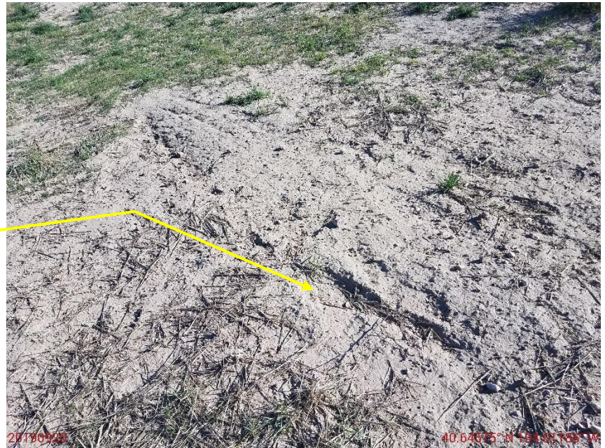
Photo 20: Continued from photo 19. Photo shows rill erosion beginning on slope.
