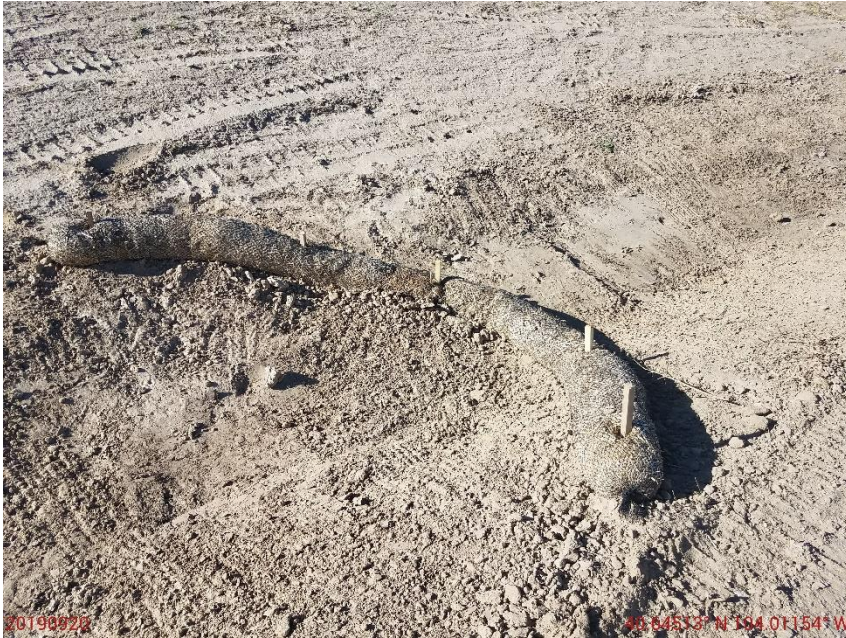
Photo 3: Photo taken from the perimeter stormwater diversion ditch. Photo shows wattles within ditch appear to have been installed in accordance with good engineering practices.
