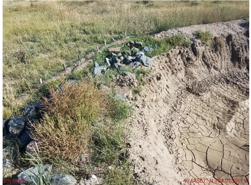
Photo 12: Photo shows outlet of the sediment trap. Outlet has not been constructed in accordance with good engineering practices.
