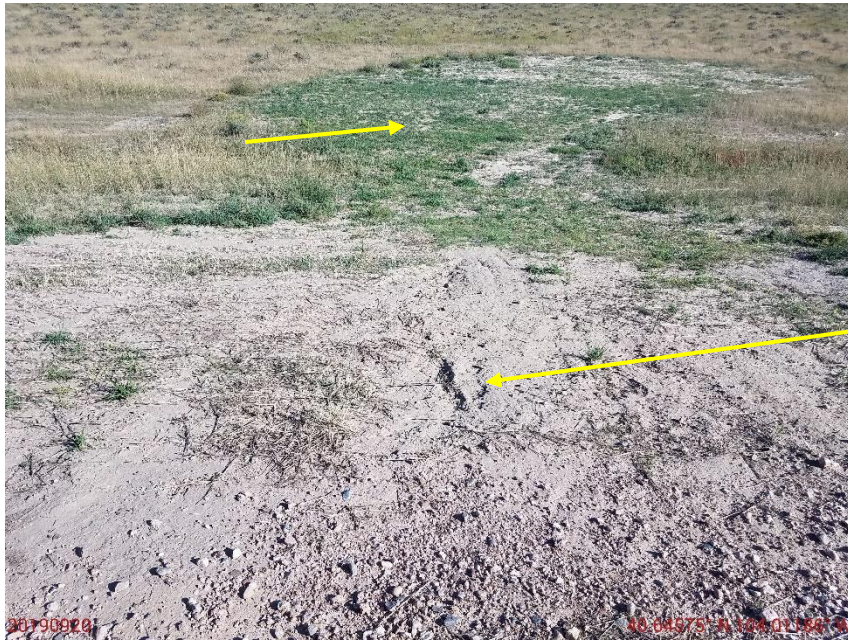
Photo 19: Photo taken from the fill slopes on the south end of the location. Photo show area where stormwater previously degraded the slope and transported sediment off location (yellow arrow). Photo also shows erosion degradation is beginning to recur along slopes. Insufficient BMPs in place to stabilize slopes.
