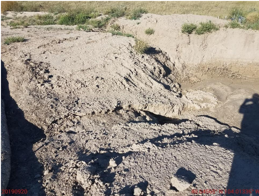
Photo 5: Continued from photo 4. Photo shows stormwater erosion degradation is beginning to recur within the trap inlet. Operator has failed to construct BMP in accordance with good engineering practices.
