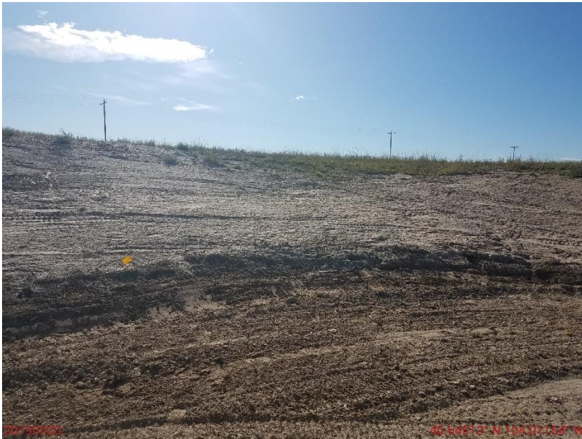
Photo 1: Photo taken from the southeast end of the location, facing southeast. Photo shows erosion degradation appears to have been repaired on the cut slopes, however, no BMPs have been installed to stabilize the slopes. Rill erosion is beginning to re-form.
