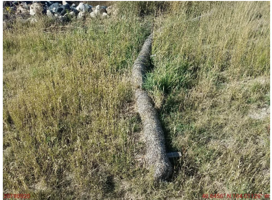
Photo 18: Photo shows straw wattle at outlet not in proper functioning condition.
