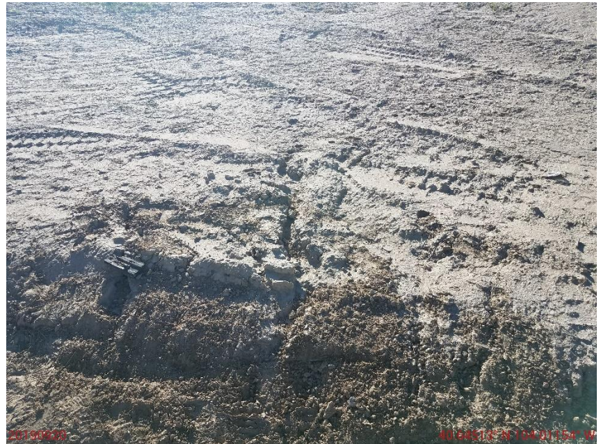
Photo 2: Continued from photo 1. Photo shows erosion degradation is beginning to recur on the cut slopes.
