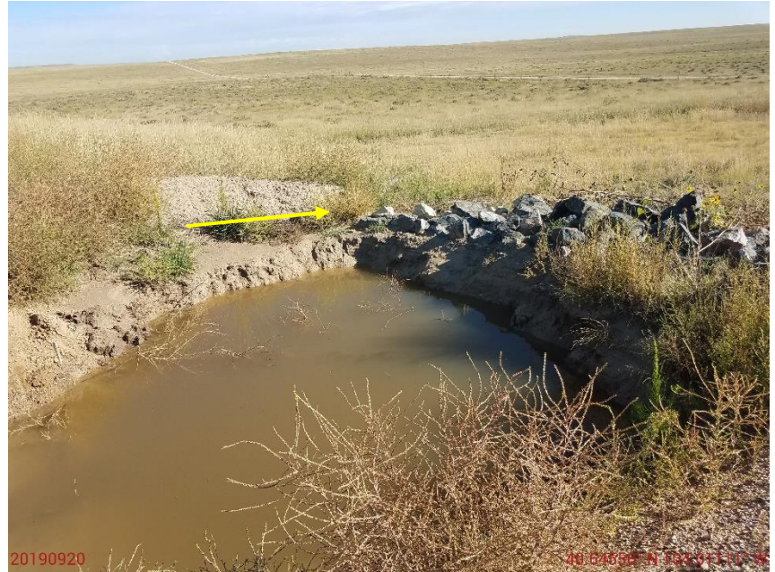
Photo 14: Continued from photo 13. Photo shows outlet at sediment trap. Outlet has not been constructed in accordance with good engineering practices.
