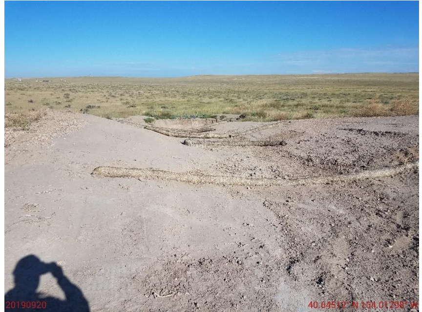
Photo 4: Photo taken from the sediment trap on the northwest end of the location, facing north. Photo shows erosion degradation appears to have been repaired. Operator appears to have re-installed wattles as inlet protection.
