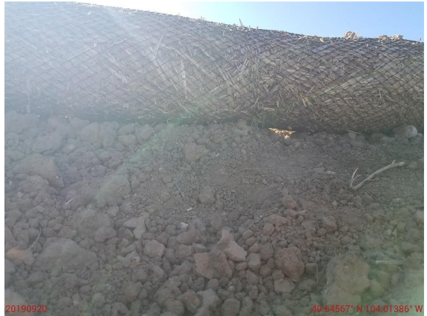
Photo 10: Photo taken from the wattle within the sediment trap inlet. Photo shows day light beneath wattle. Insufficient inlet protections at sediment traps.
