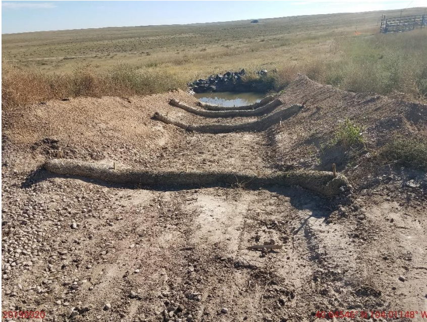
Photo 13: Photo taken from the sediment trap on the northeast end of the location, facing east. Photo shows erosion degradation appears to have been repaired at inlet. Operator appears to have re-installed wattles as inlet protection.
