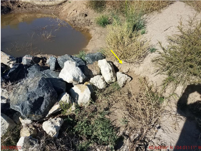
Photo 15: Continued from photo 14. Photo shows outlet has not been constructed in accordance with good engineering practices. Stormwater movement around outlet and degradation evident
