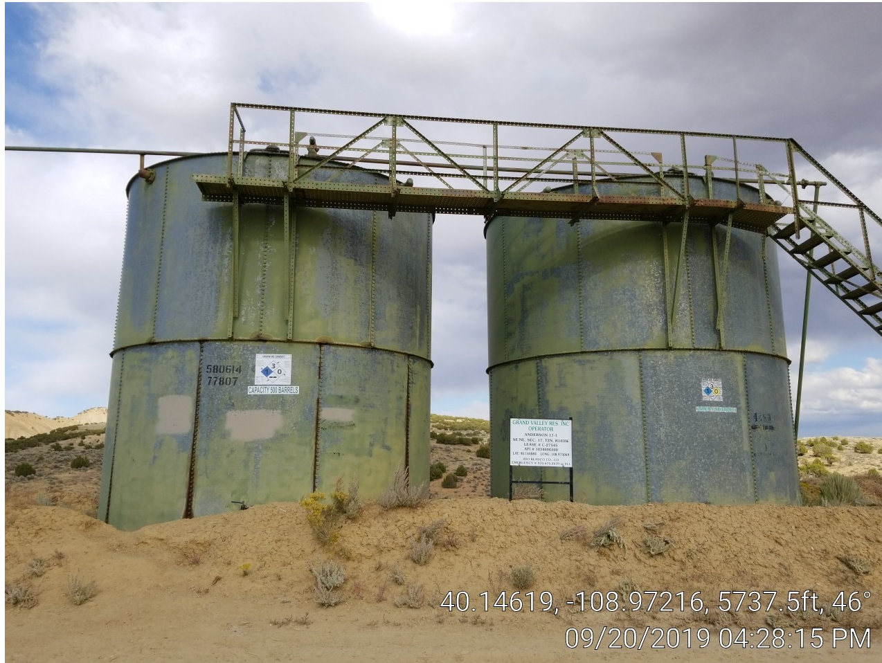
Photo 1. Tank battery.
