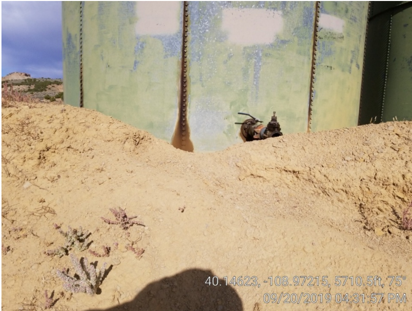
Photo 5. Low spot in tank berm.
