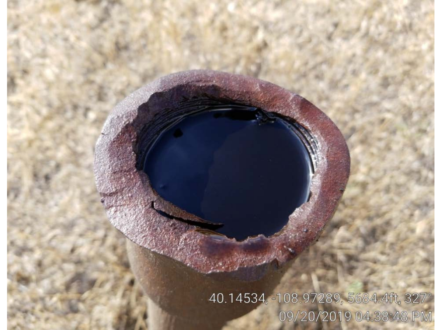
Photo 8. Flowline filled with oil to top.
