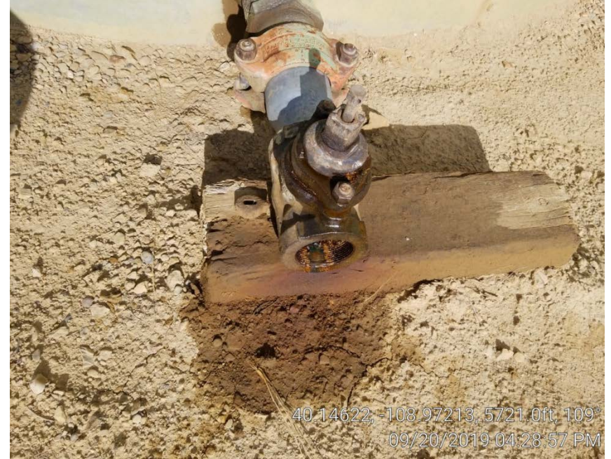
Photo 4. Stained soil at crude oil tank valve.
