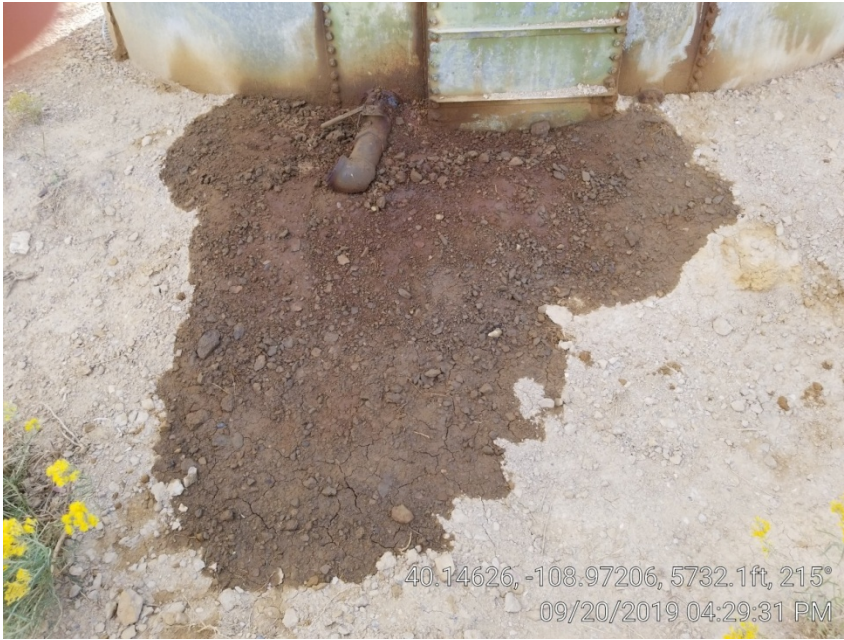
Photo 3. Stained soil at crude oil tank valve.
