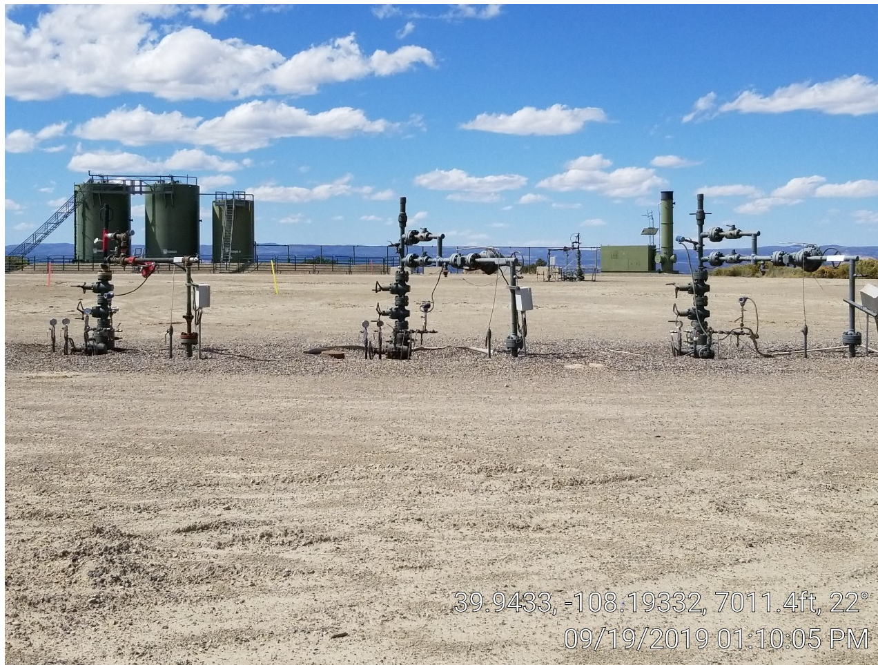
Photo 1. Wells, tanks battery, and separator.
