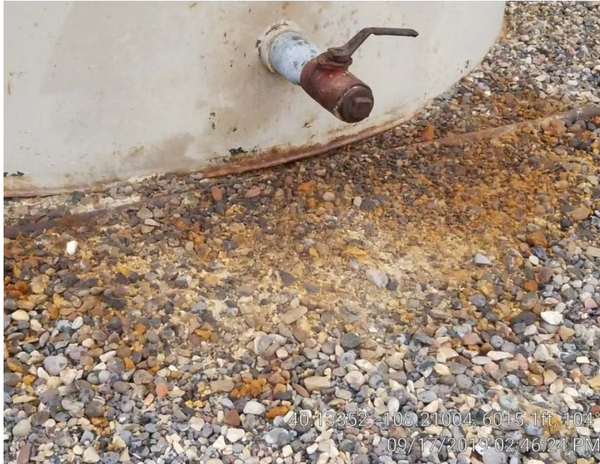
Photo 2. Stained gravel next to water tank.
