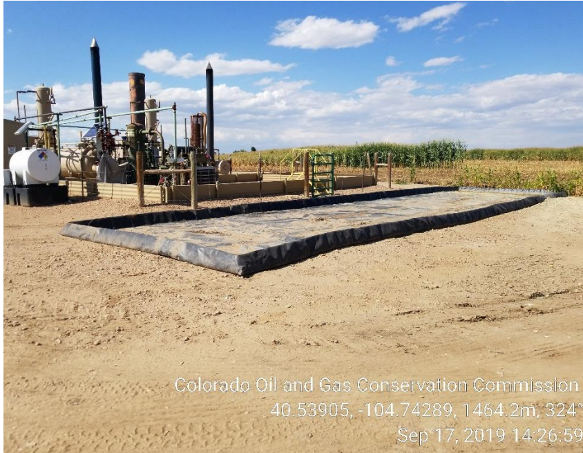
Photo 5: Unused secondary containment device on location
