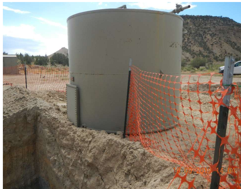
Photo #10 – View of inadequate berms around the 100 BBL AST.
