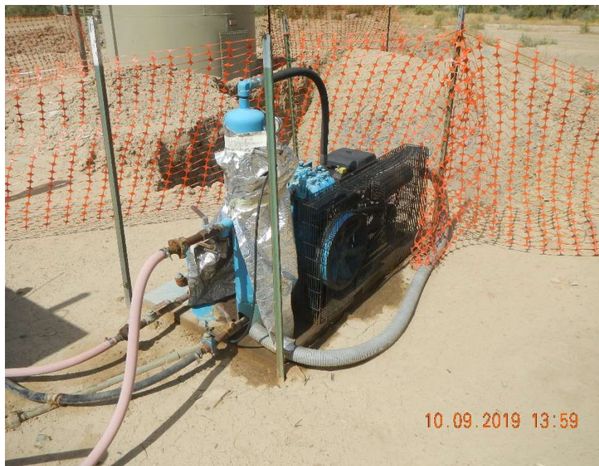
Photo #9 – View of stained soil beneath the compressor unit.
