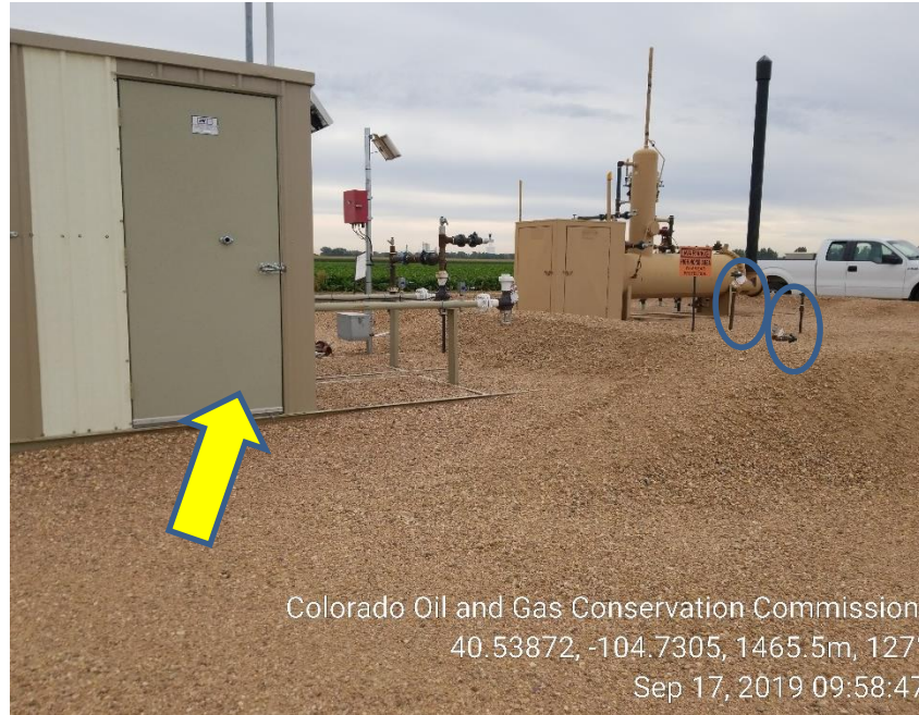
Photo 5: Disconnected gas meter house, Unused risers
