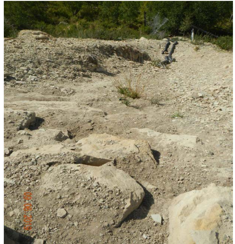
Photo#5: Views of un-stabilized overly Steep Fill Slopes.
