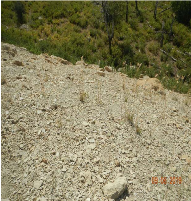
Photo#4: Views of un-stabilized overly Steep Fill Slopes.
