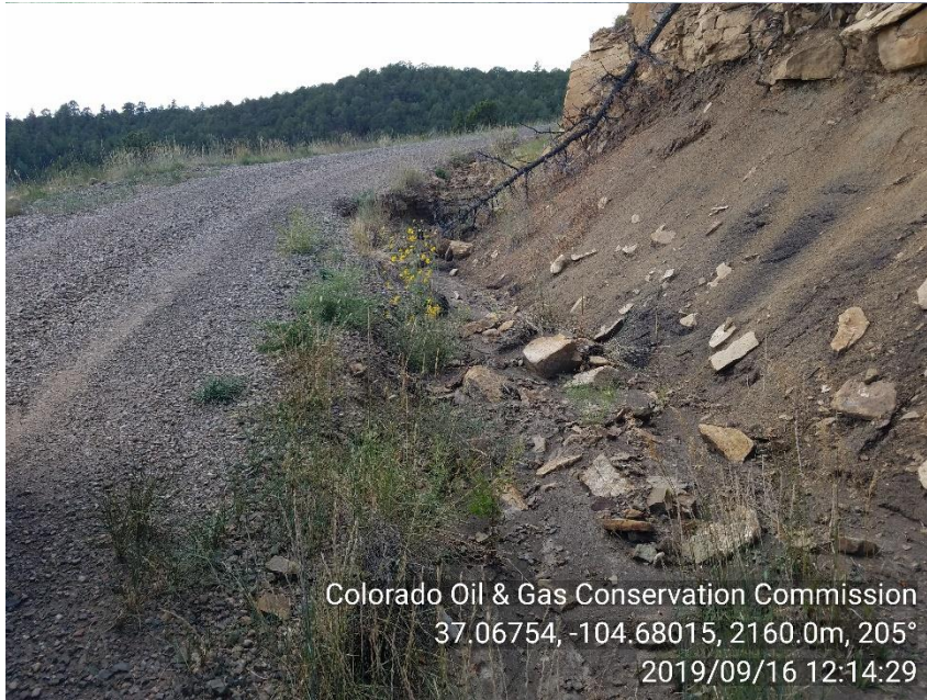
PHOTO 9: EROSION IN BMP DITCH ALONG ROW NORTHWEST OF LOCATION. REPAIR EROSION AND INSTALL ADEQUATE BMP'S TO PREVENT OR REDUCE EROSION, COMPLY WITH RULE 1002.f. CA DATE 10-16-19
