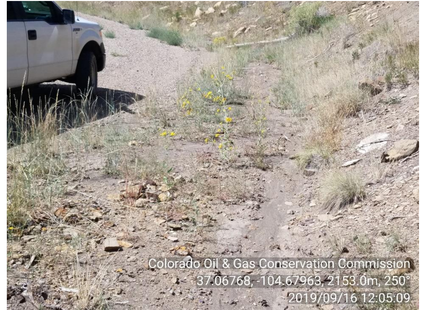
PHOTO 4: THIS IS THE CURENVT PHOTO AND CORECTIVE ACTION FOR THIS INSPECTION. SEDIMENT HAS FILLED STORMWATER DRAIN ON UPSLOPE SIDE OF PLUGGED CULVERT. CLEAN AND MAINTAIN BMP DITCH PER RULE 1002.f. CA DATE 10-16-19
