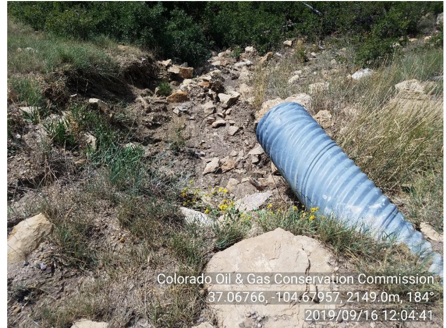
PHOTO 6: THIS IS A CURRENT PHOTO AND CA FOR THIS INSPECTION. STORMWATER EROSION AROUND CULVERT OUTLET. Install or repair required BMPs per Rule 1002.f. CA DATE IS IMMEDIATELY BEGIN WORK TO REPAIR EROSION.
