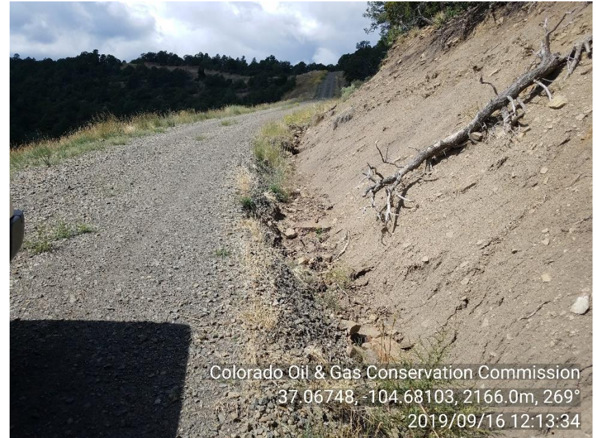
PHOTO 10: EROSION IN BMP DITCH ALONG ROW NORTHWEST OF LOCATION. REPAIR EROSION AND INSTALL ADEQUATE BMP'S TO PREVENT OR REDUCE EROSION, COMPLY WITH RULE 1002.f. CA DATE 10-16-19
