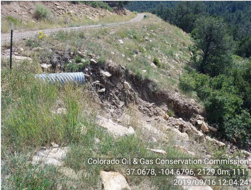
PHOTO 7: ANOTHER VIEW OF EROSION AROUND CULVERT OUTLET.
