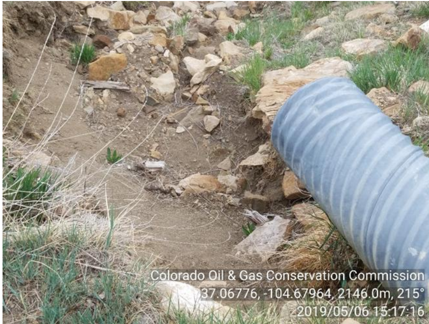
PHOTO 5: THIS IS A PHOTO AND CORRECTIVE ACTION FROM PREVIOUS INSPECTION DOC#695100599. STORMWATER EROSION AROUND CULVERT OUTLET. Install or repair required BMPs per Rule 1002.f
