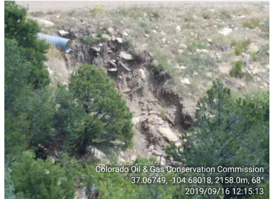
PHOTO 8: ANOTHER VIEW OF EROSION AROUND CULVERT OUTLET.
