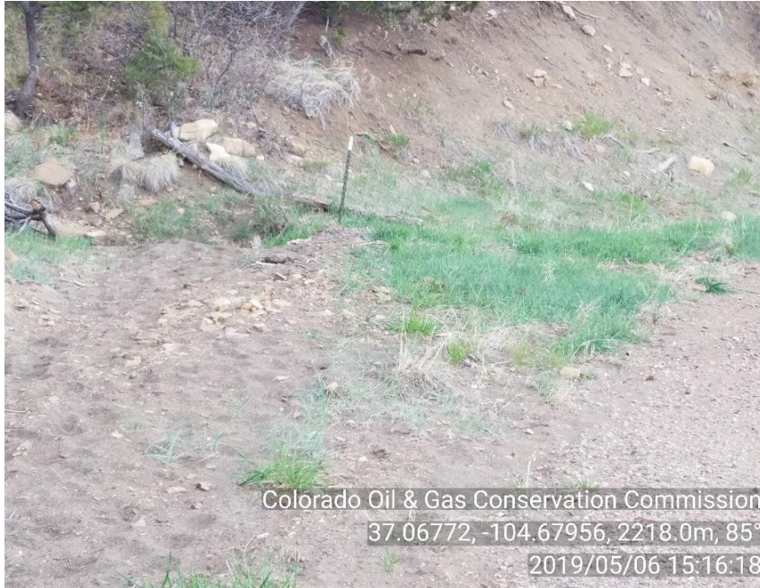
PHOTO 3: THIS IS A PHOTO AND CORRECTIVE ACTION FROM PREVIOUS INSPECTION DOC#695100599. SEDIMENT HAS FILLED STORMWATER DRAIN ON UPSLOPE SIDE OF PLUGGED CULVERT
