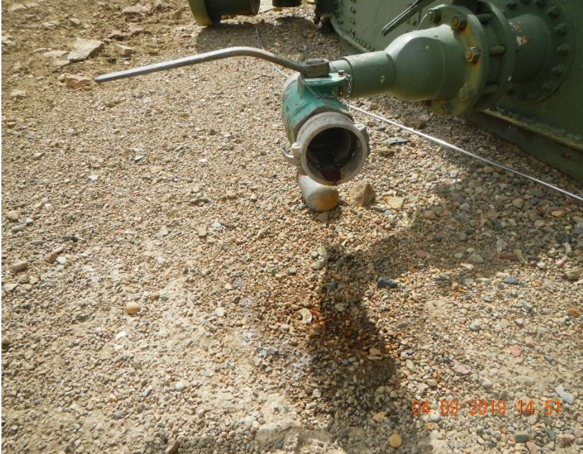
Photo #3 – View of active drip coming from the 2000 BBL produced water AST.
