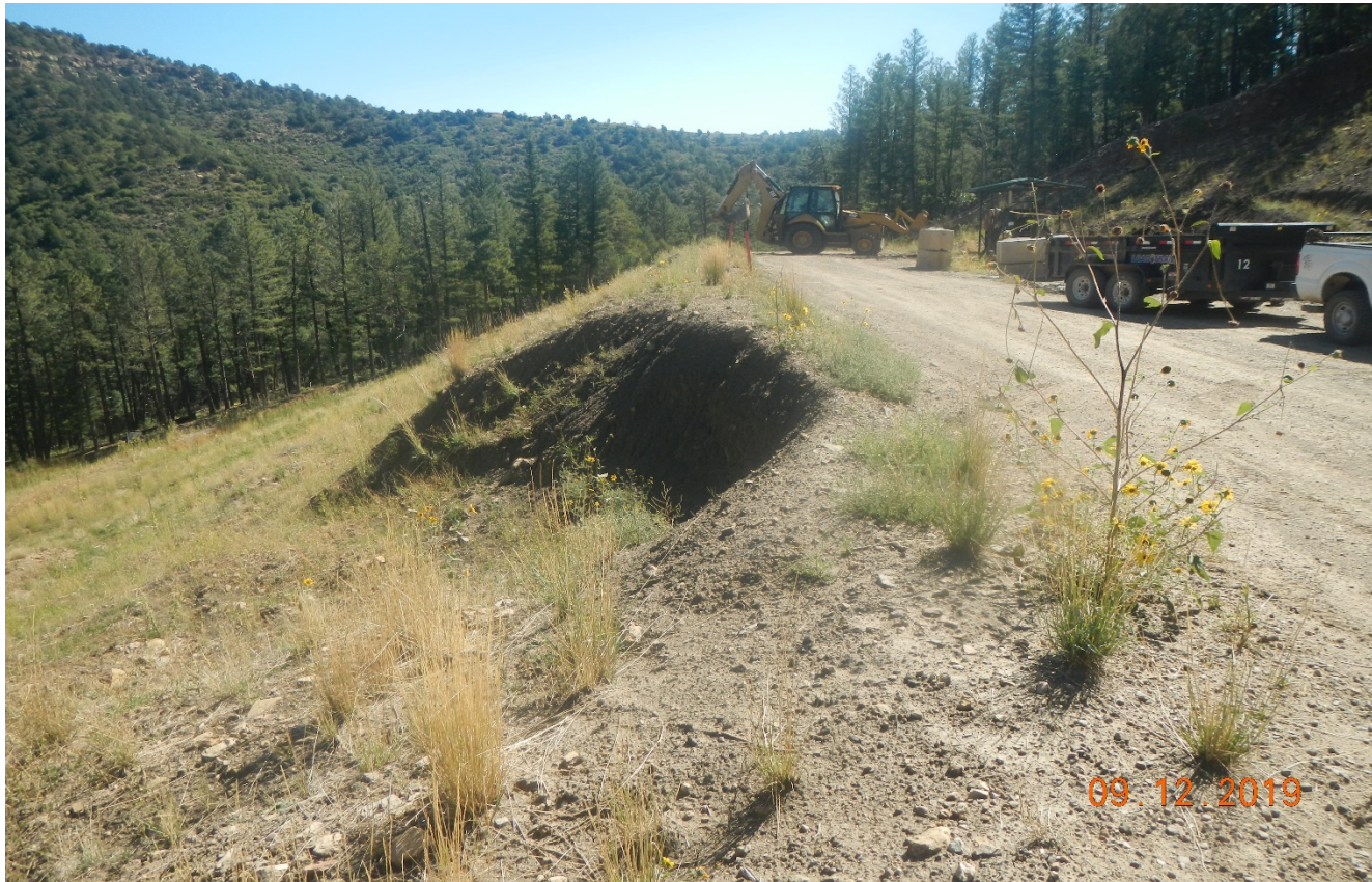
Photo 1. There is soil sloughing that occurred at the east side of the location. Corrective action of the previous inspection was not performed.
