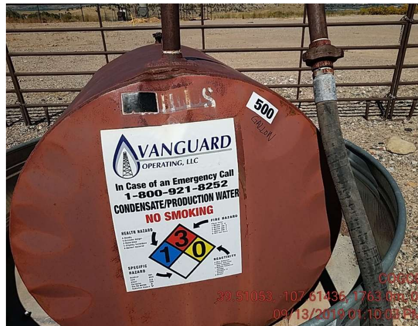
Tank labeled with capacity by pumper on location
