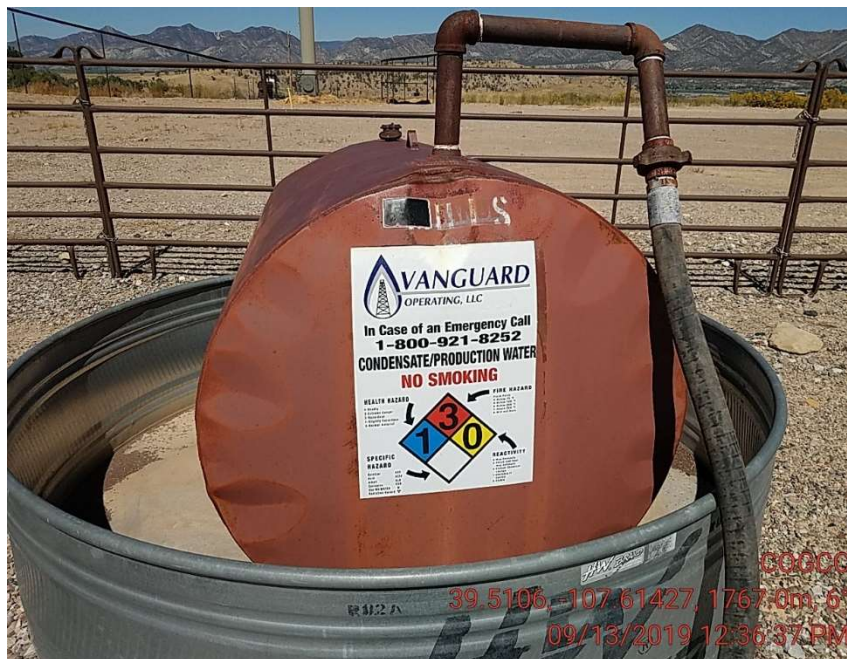
Tank not labeled with capacity
