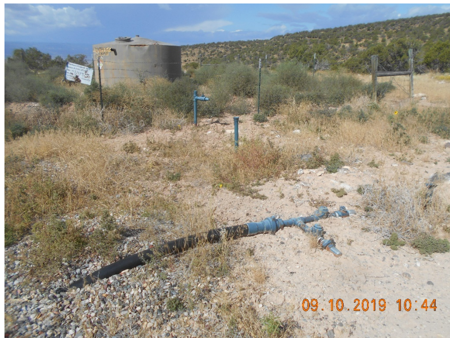
Unused 2" risers and 4" off location flowline. Bullplugs in flowline and 1 riser. 1 Riser open ended.
