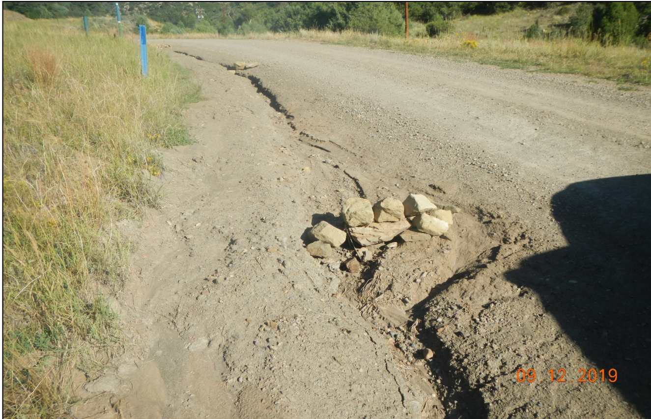
Photo 3. The rock check dams were not installed correctly. Stormwater is flowing around the checkdams causing erosion of the road.
