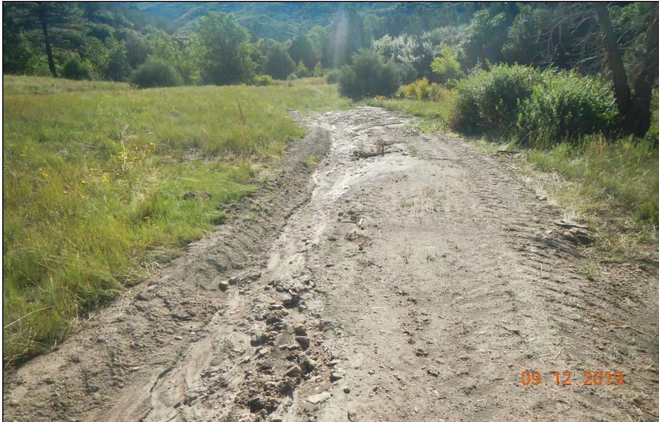
Photo 2. Sediment has already filled into the diversion ditch since grading occurred. No work has been conducted here since previous inspection. Erosion must be controlled to prevent sediment discharge. This area of disturbance needs to be seeded and stabilized.
