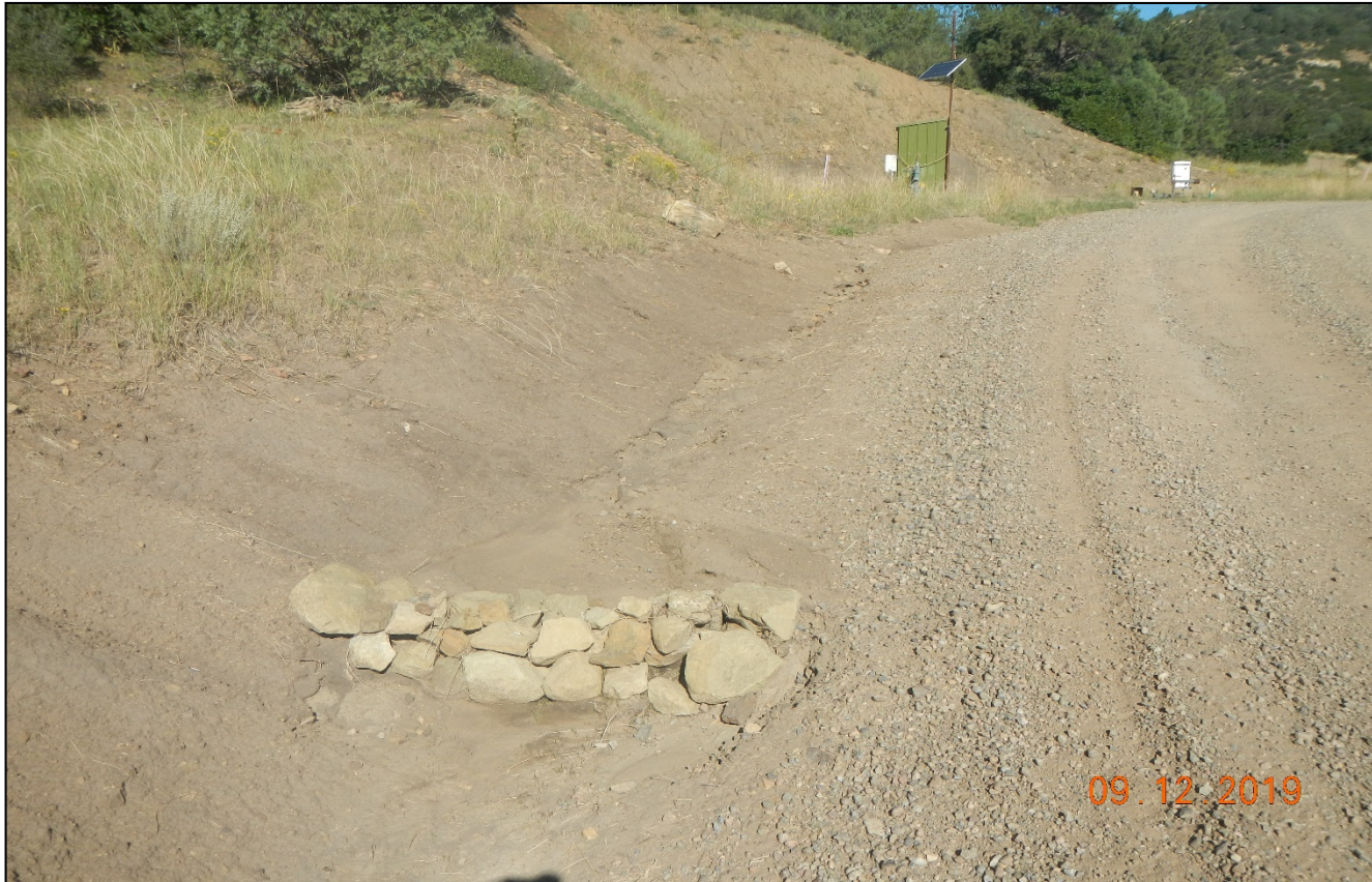
Photo 5. Photo of another checkdam further along the road. The rock check dam has filled in with sediment. Erosion needs to be controlled from the source.
