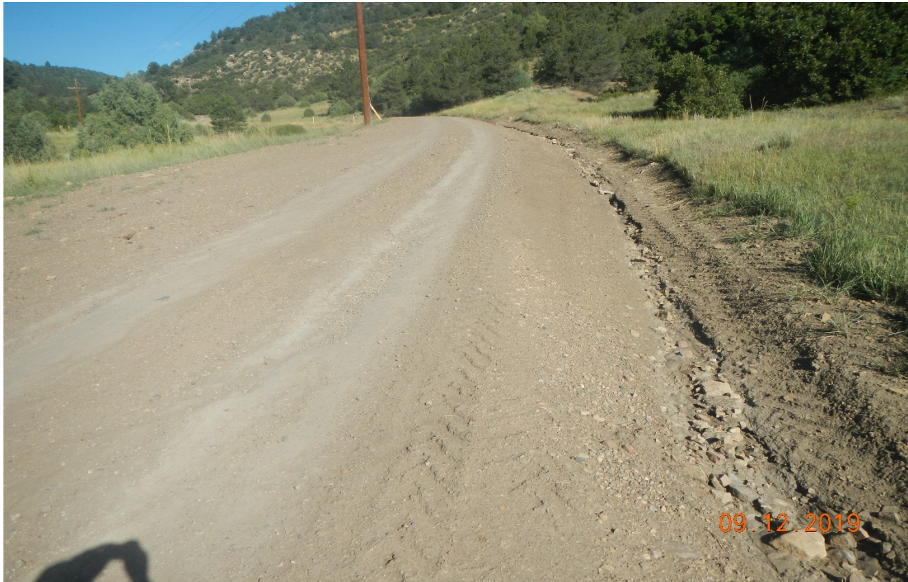
Photo 1. Facing northwest near the mouth of the canyon. The main road has recently be graded. Erosion is occurring along the side of the road.
