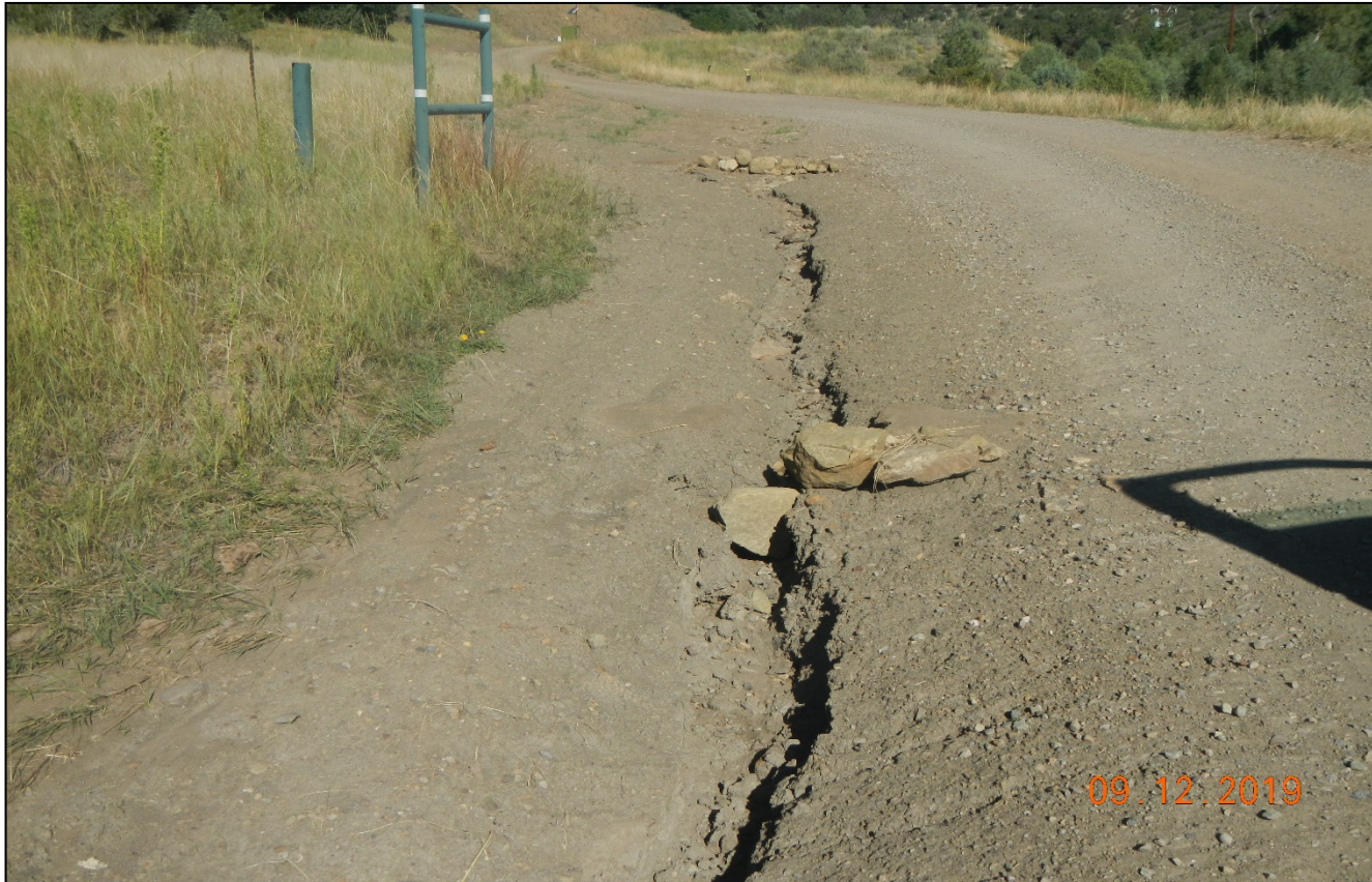
Photo 4. Photo of another checkdam further along the road. The rock check dams were not installed correctly. Stormwater is flowing around the checkdams causing erosion of the road.
