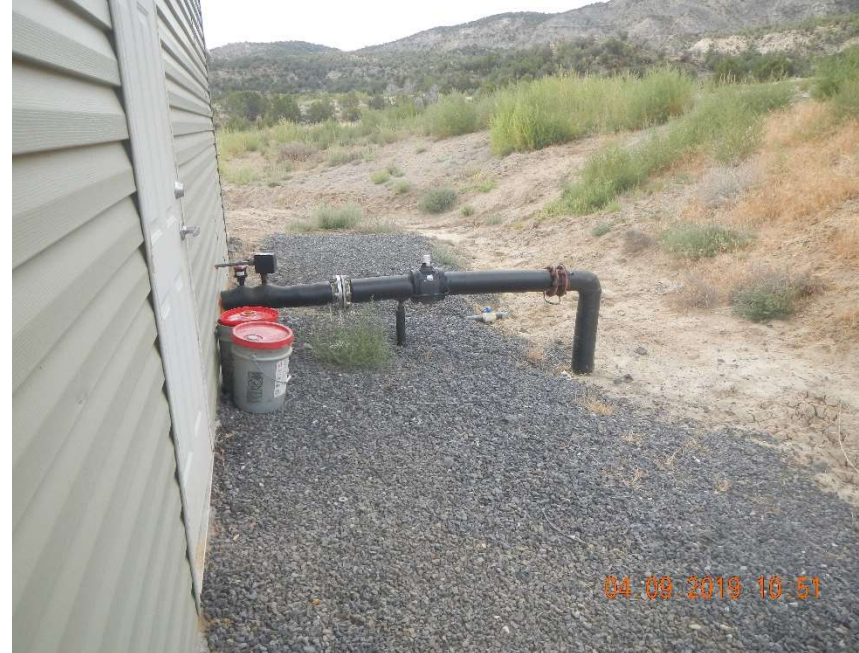
Photo #6 – View of the 3-inch and 2-inch flowline on the west side of the pump house.
