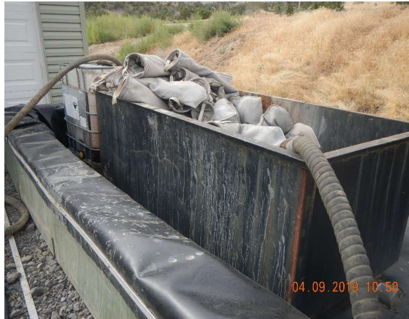
Photo #11 - Photos of filter socks and poly cube tank within secondary containment.
