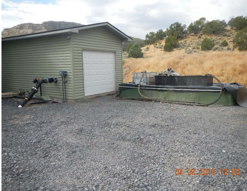
Photo #5 – View of the pump house, the 3-inch and 4-inch flowline on the east side of the building, and the lined containment area with the filter socks and poly cube container.
