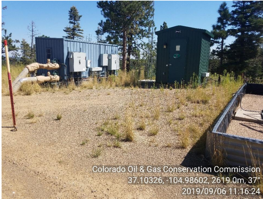
PHOTO 5: WEEDS AROUND TANK BATTERY CONTAINMENT. CUT WEEDS AND MAINTAIN WEEDS AROUND EQUIPMENT IN ACCORANCE WITH RULE 603.f. CA DATE 10-6-19
