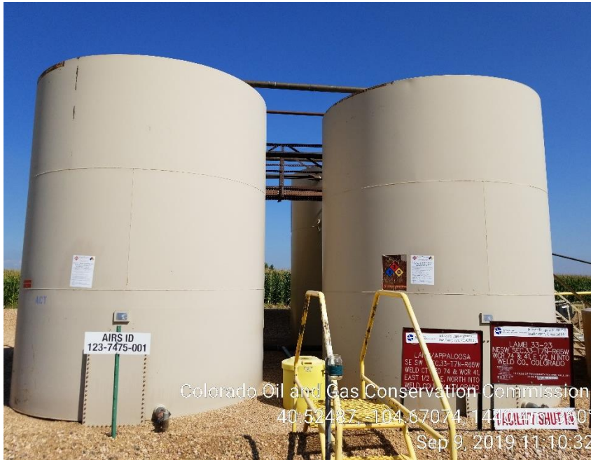
Photo 5: No Labeling on North tanks
