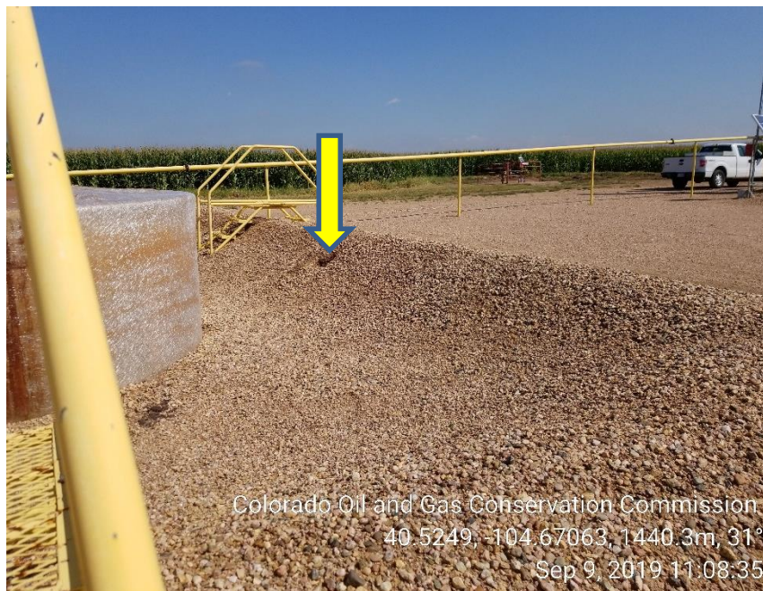
Photo 9: Hole in tank battery (east) berm wall.
