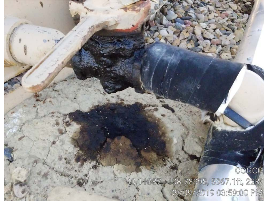
Photo 16. Crude oil tank valve.
