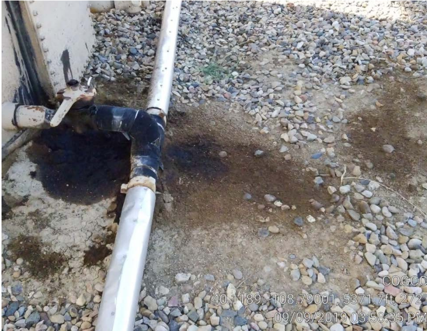
Photo 15. Crude oil tank valve.
