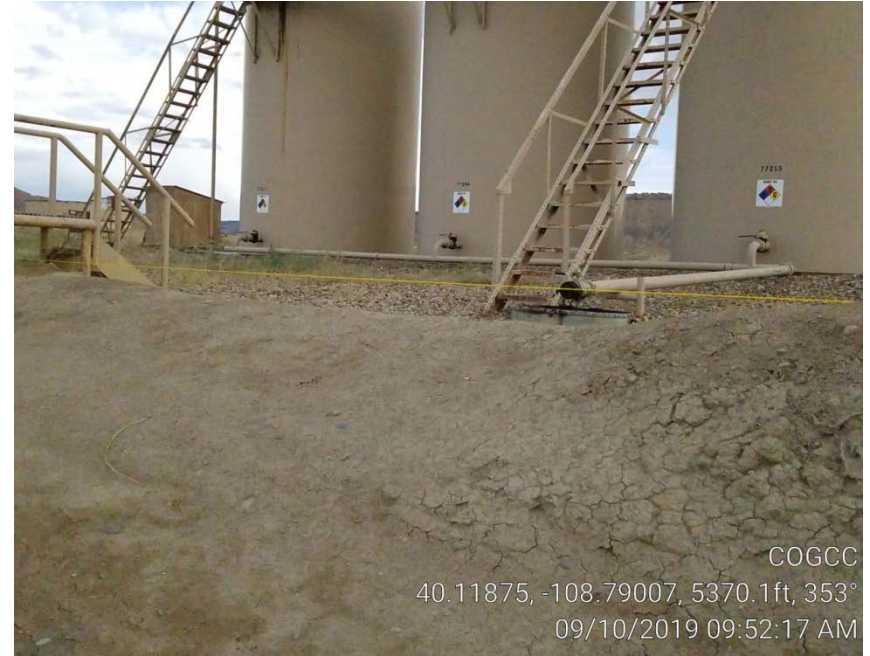
Photo 10. Berm height too short for crude tanks.
