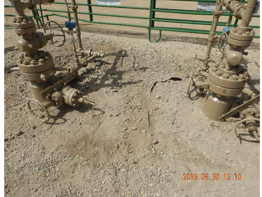
Photo #4 – Close-up view of backfilled well cellars.
