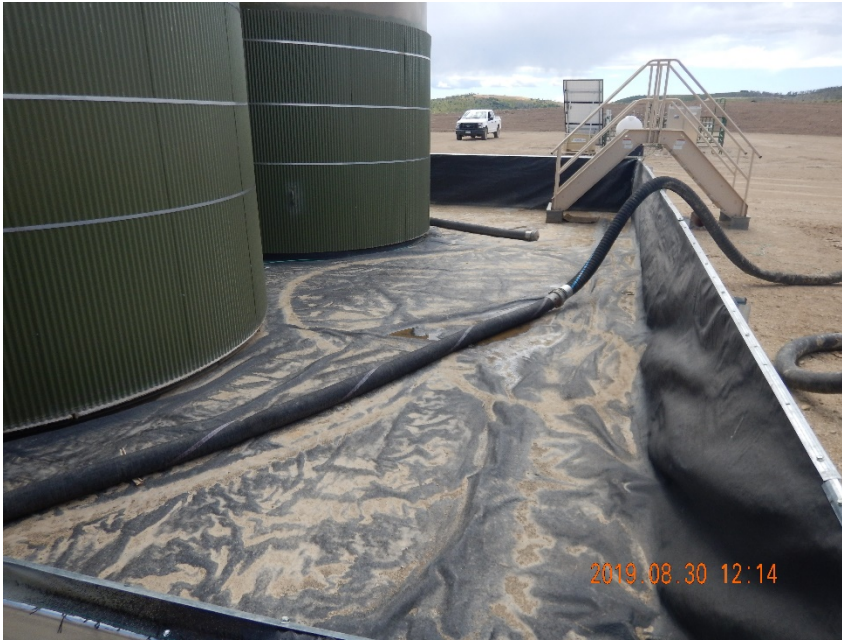
Photo #7 – Hoses stored on west side of tank battery secondary containment with metal fittings in direct contact with liner.
