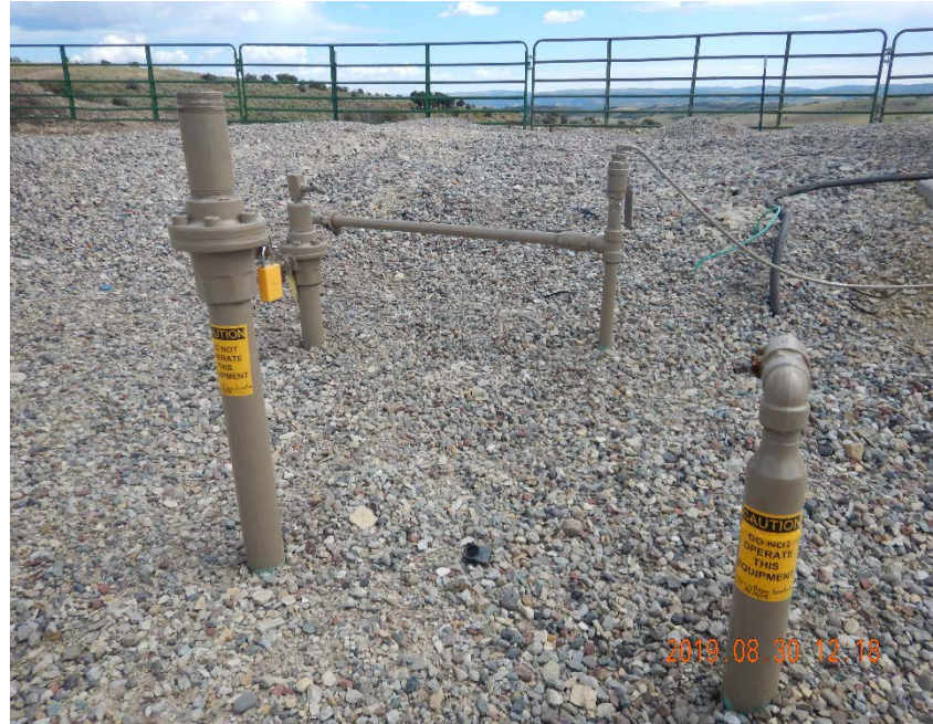
Photo #11 – Flowline risers north of separators have been LO/TO.
