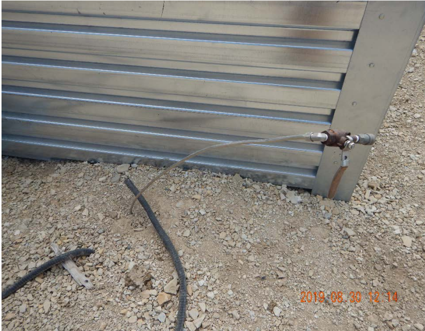
Photo #9 – Unused, unmarked, and uncapped ¼" riser located northwest of tank battery. Operator was instructed to LO/TO and remove this riser in previous FIR (doc #690200036).
