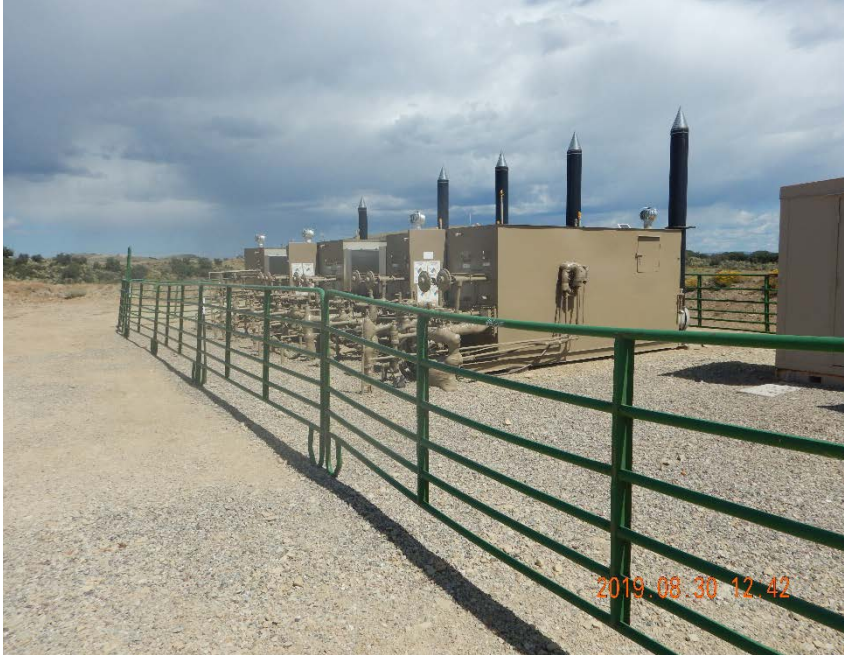
Photo #7 – Heated horizontal separators on east side of location.
