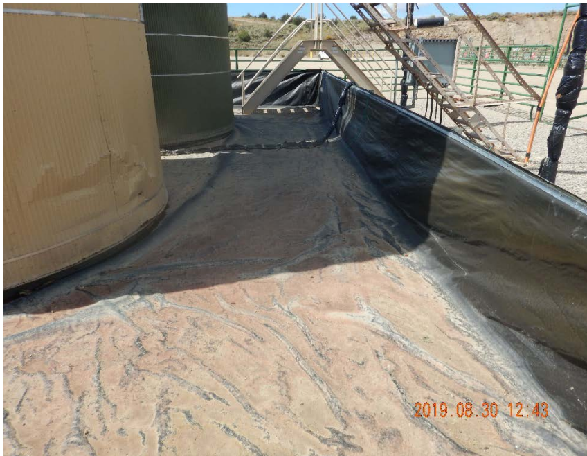
Photo #9 – View of lined tank battery secondary containment area (north side).
