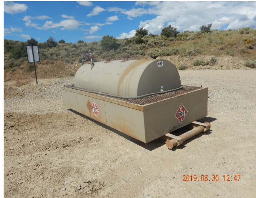
Photo #10 – Diesel AST with secondary containment device located on west side of location.
