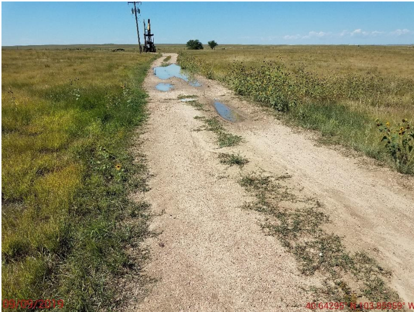
Photo 1: Photo taken from the access road, facing west. Photo shows that access road has not been constructed or sufficient BMPs installed to allow for proper stormwater discharge to ensure existing access road remains in proper functioning condition.
