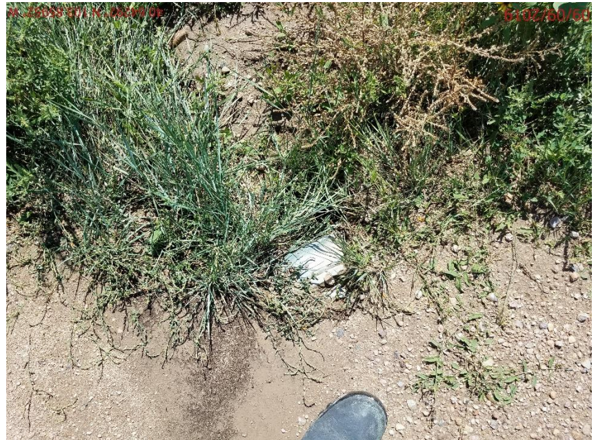
Photo 2: Photo shows culvert at access road is not longer in proper functioning condition.
