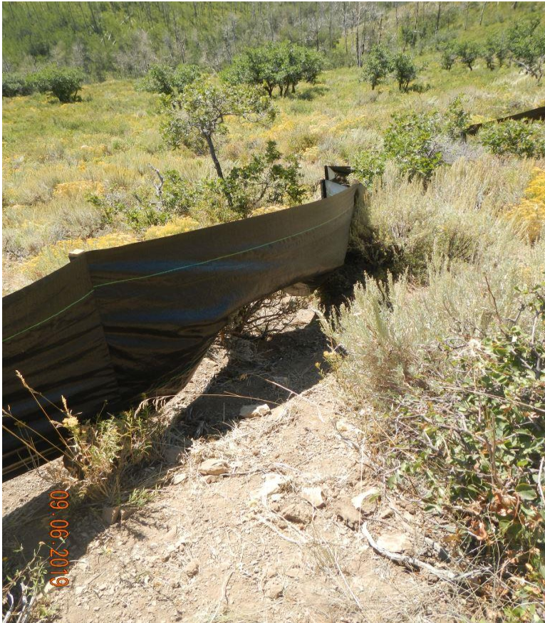
Photo#2: Silt fence is not Properly installed.
