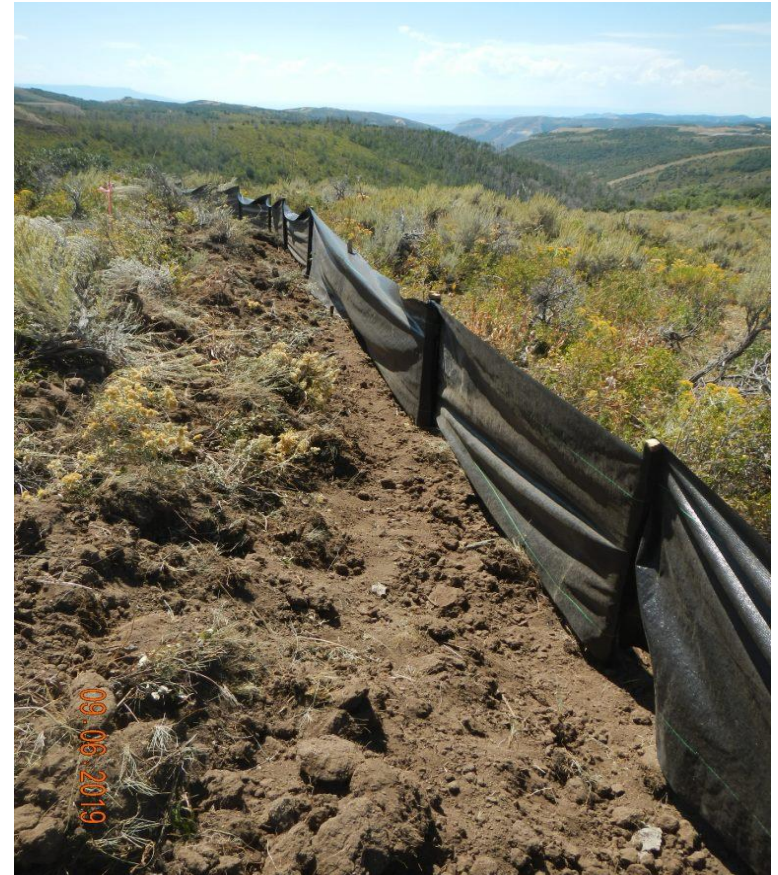
Photo#3: Silt fence is not Properly installed.
