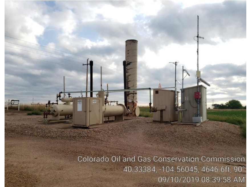
Photo #2 Separator, ECD, & Meter Runs
