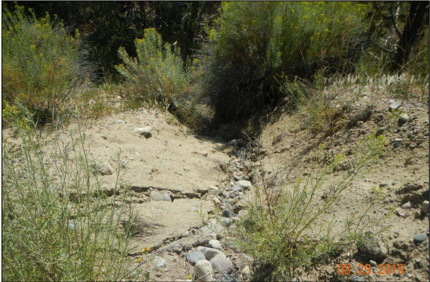
Photo 4. View of erosional channel within the eastern project area. Cobbles in channel are not adequate stormwater controls.
