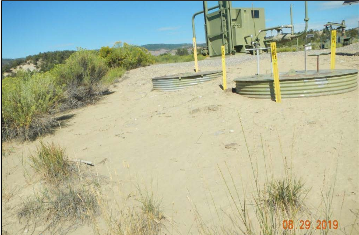
Photo 3. View of bare and unstabilized soils within the southeastern project area. Stabilization/revegetation is needed here.
