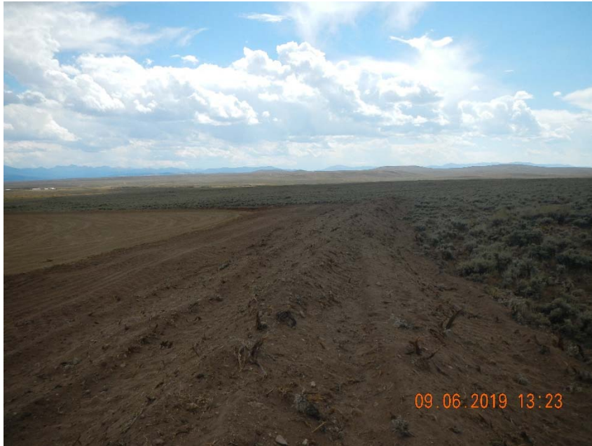
Photo 5. Possible topsoil. No stormwater controls or topsoil protections apparent.
