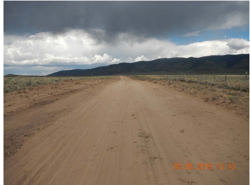
Photo 12. Access road with no stormwater controls apparent.
