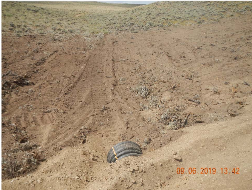
Photo 11. No stormwater controls apparent in drainage crossing.
