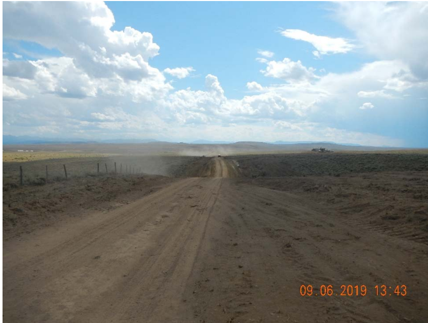
Photo 9. Access road before drainage crossing. Dust from contractors vehicles and my own vehicle visible in photo. No stormwater controls apparent.
