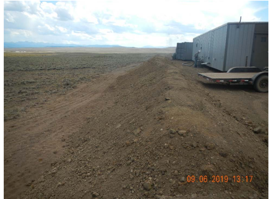
Photo 2. Non-compacted perimeter berm, no stormwater controls apparent.
