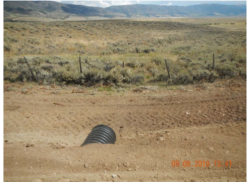
Photo 10. No stormwater controls apparent in drainage crossing.
