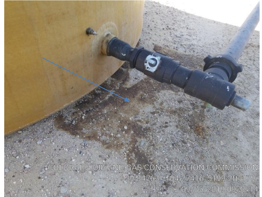
Pic 12 stained soil/mechanical conditions
