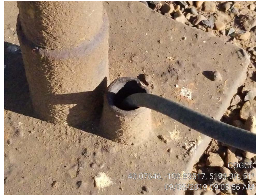
Photo 3. Casing open to atmosphere.
