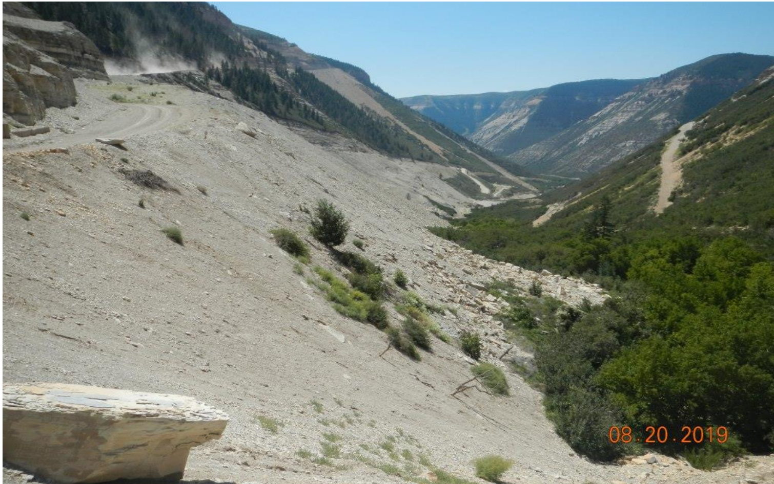
Photo#2: Access road fill slope is unstable.
