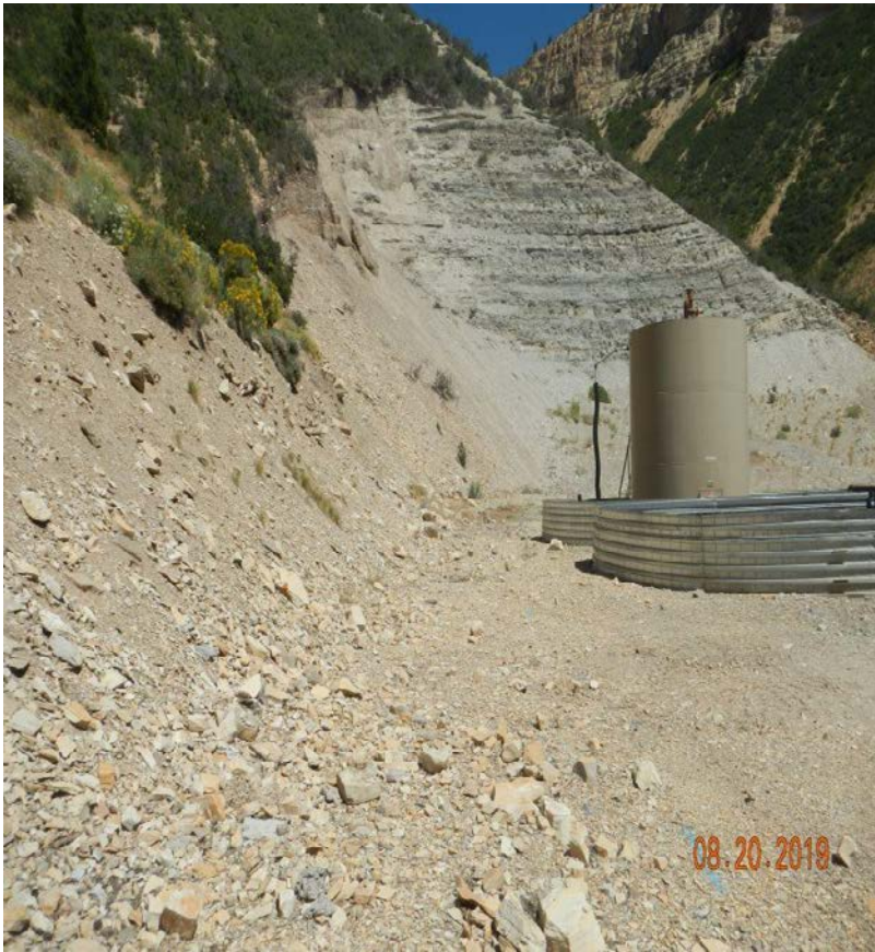
Photo#3: Further stabilization of Cut slopes is needed
