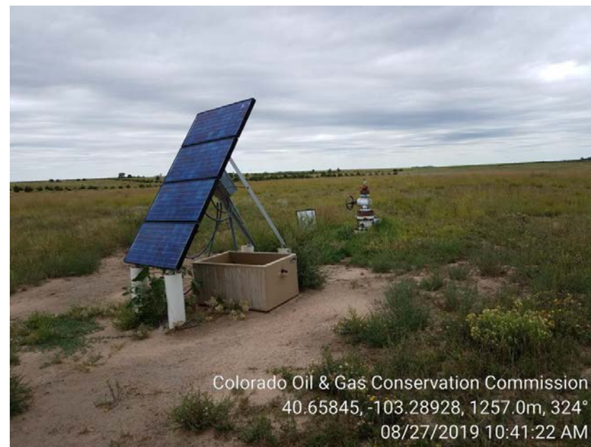
2. Wellhead, Solar powered cathodic rectifier
