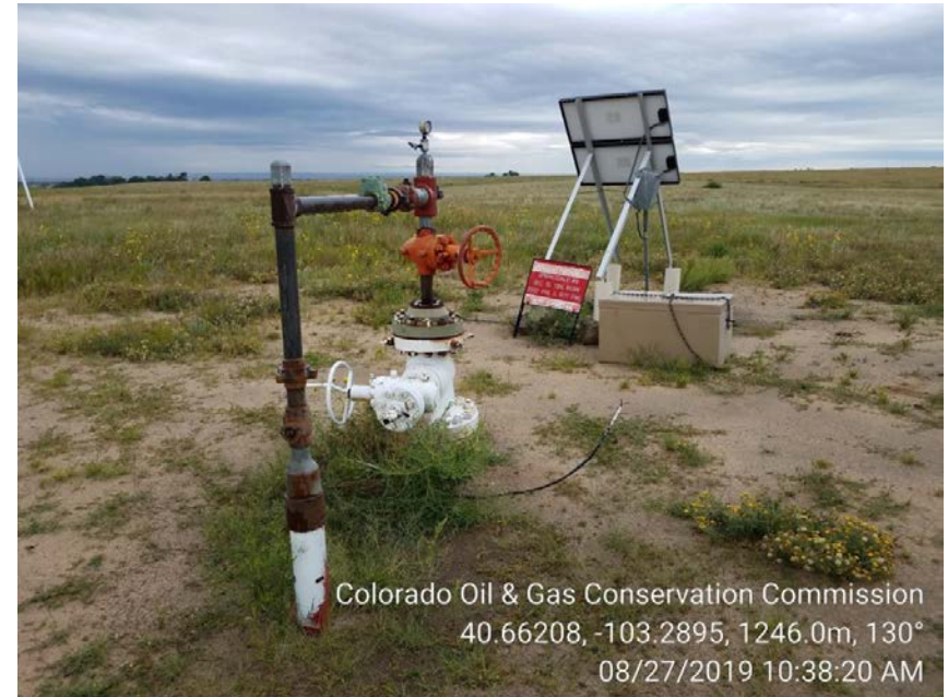
2. Wellhead, Solar powered cathodic rectifier
