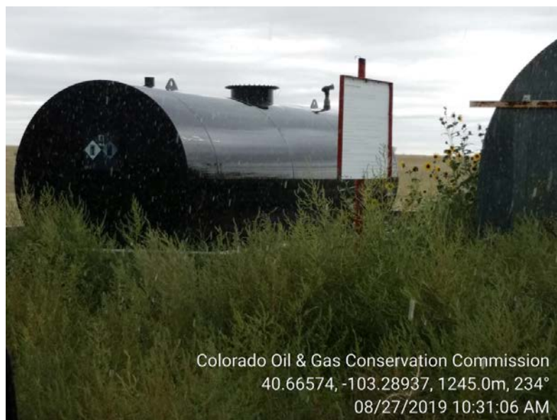
3. Free water knockout and weeds
