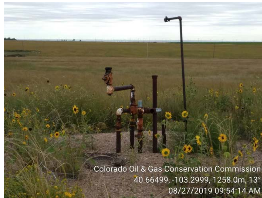
6. Unmarked or locked out production risers
