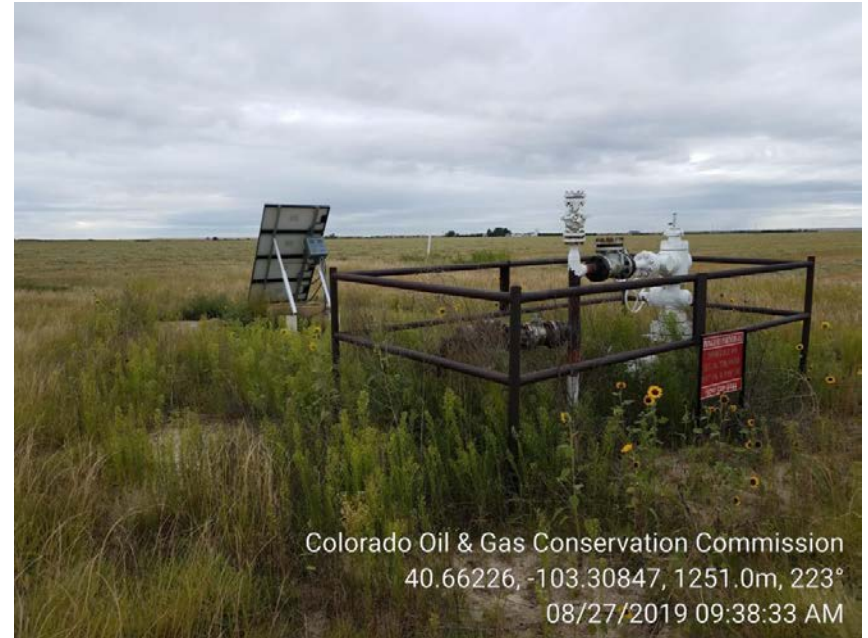
2. Wellhead, solar powered cathodic rectifier and vegetation
