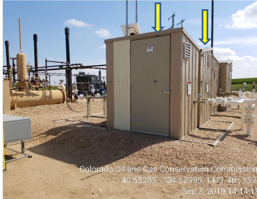
Photo 7: Disconnected gas meter houses.
