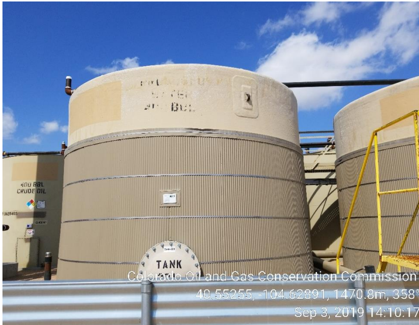
Photo 5: Produced water tank missing labeling.
