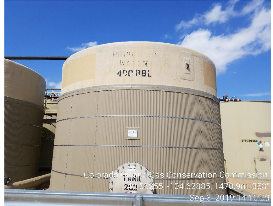
Photo 4: Produced water tank faded labeling
