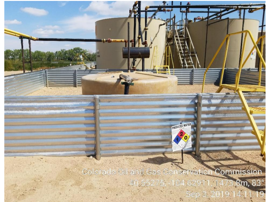
Photo 6: Missing labeling on produced water tank
