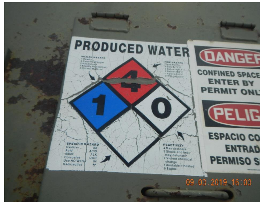
200 bbl tank Produced water label is damaged.
