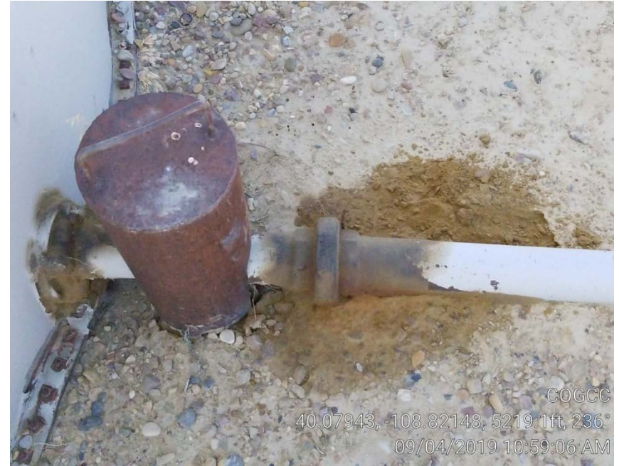
Photo 7. Stained soil next to tank.
