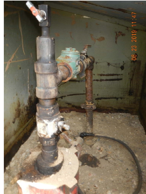
Photo 2. Photo of wellhead inside housing, stained soil at wellhead.
